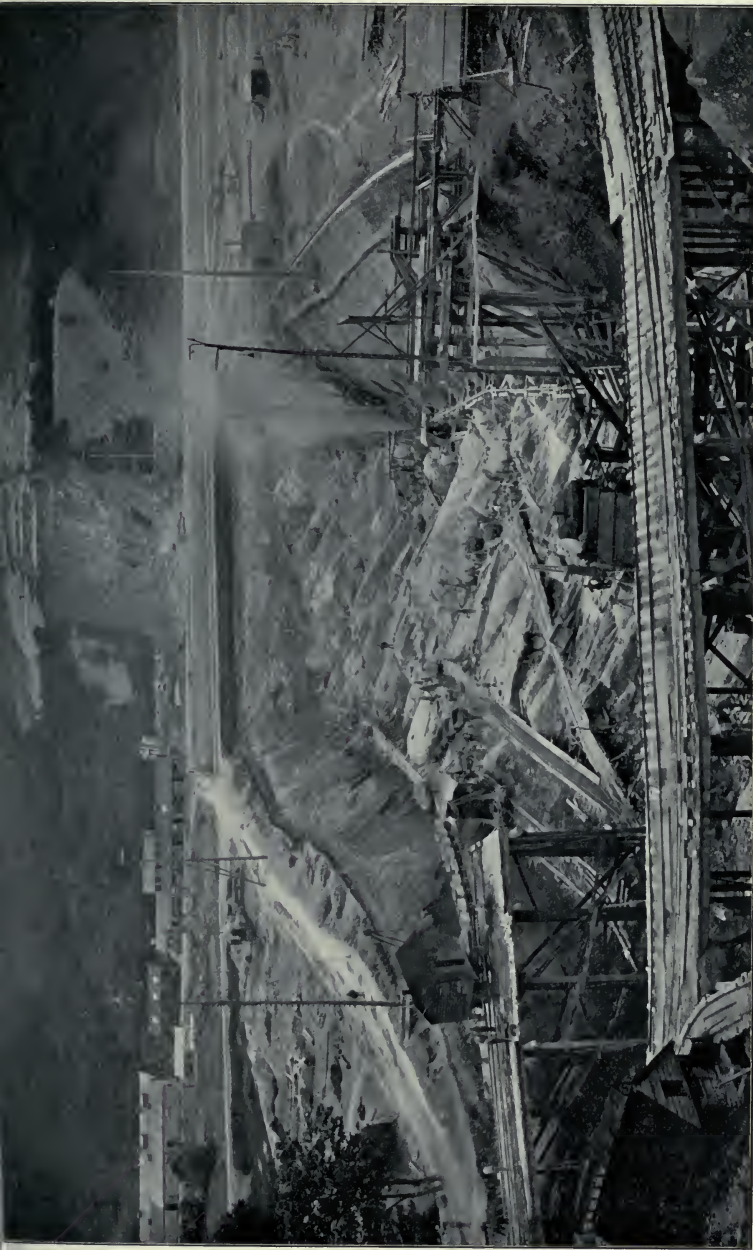
No. 1. THE VYRNWY DAM—EXCAVATING THE TRENCH ACROSS THE VALLEY OF THE RIVER VYRNWY.
