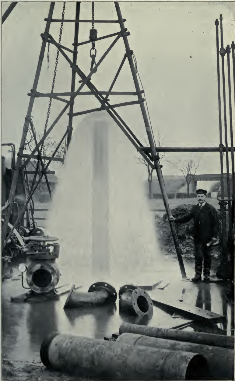
A TYPICAL ARTESIAN BORING.
