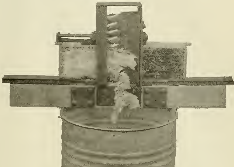
NO. 2—FERGUSON UNCAPPING MACHINE—SIMPLER ADJUSTMENT.
