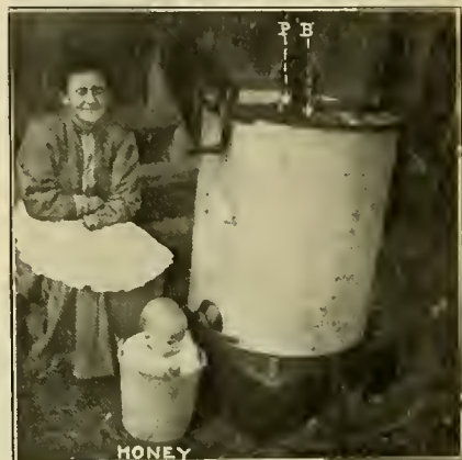
FIG. 1.—HONEY-EXTRACTOR READY FOR OPERATION.
