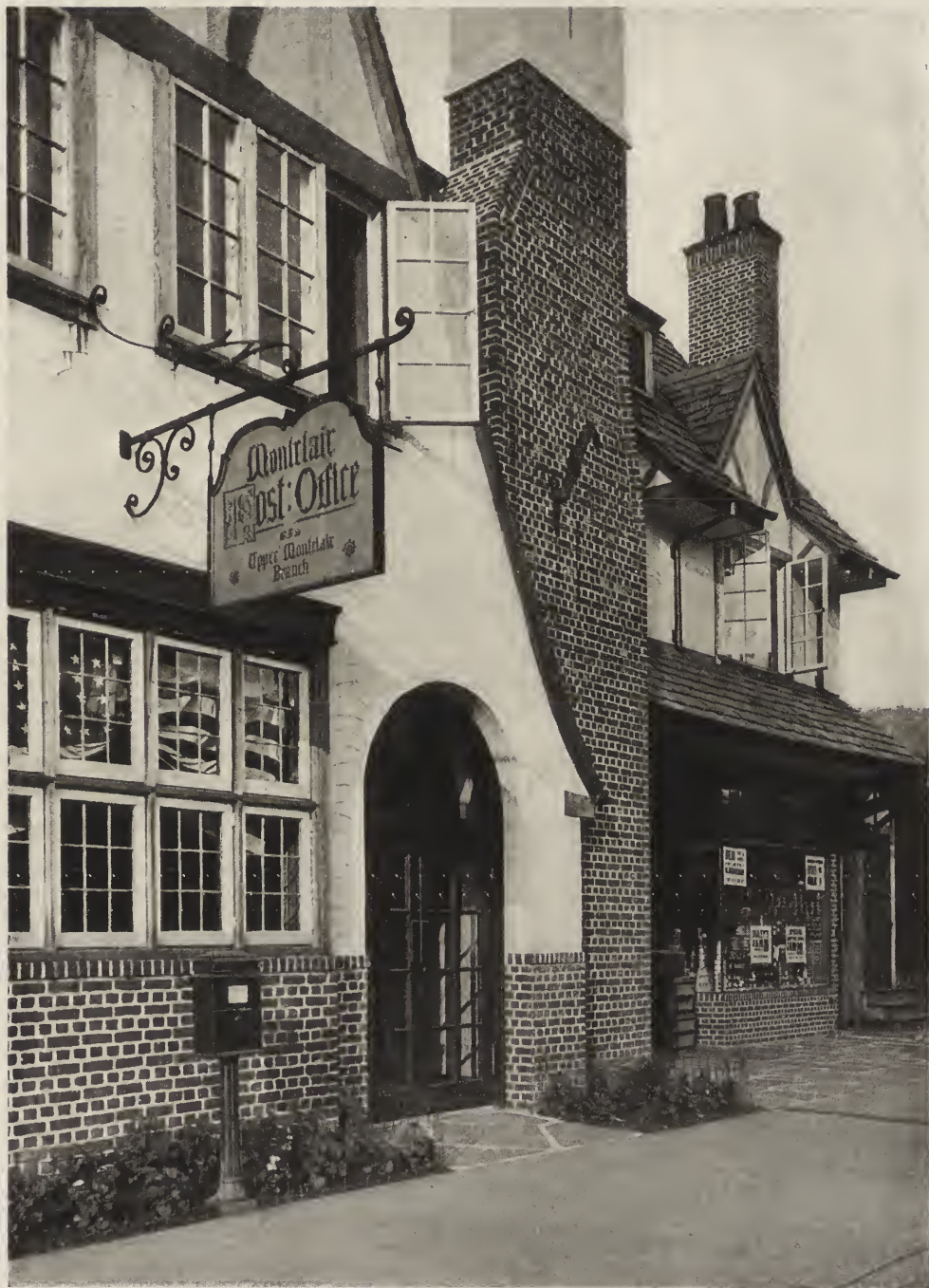
DETAIL OF POST OFFICE, UPPER MONTCLAIR, N. J. FRANCIS A. NELSON, ARCHITECT.
