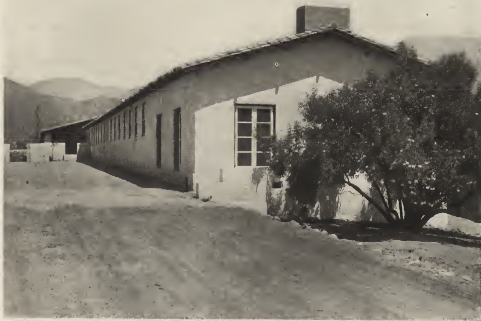
VIEW FROM THE SOUTH—FLINTRIDGE COUNTRY CLUB, FLINTRIDGE, NEAR PASADENA, CAL. Myron Hunt, Architect
