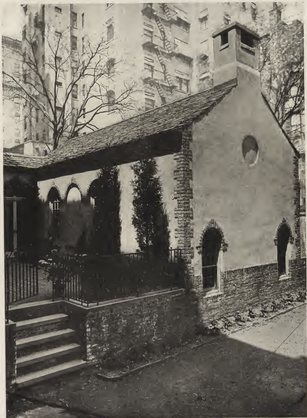
TROPHY ROOM (BEYOND DINING ROOM GARDEN)—RESIDENCE OF BAYARD DOMINICK, ESQ., 115-117 EAST 54TH STREET, NEW YORK CITY. WILLIAM F. DOMINICK, ARCHITECT.
