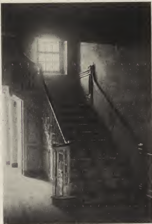
STAIRWAY IN KEEPER'S HOUSE, CHARMING FORGE.
