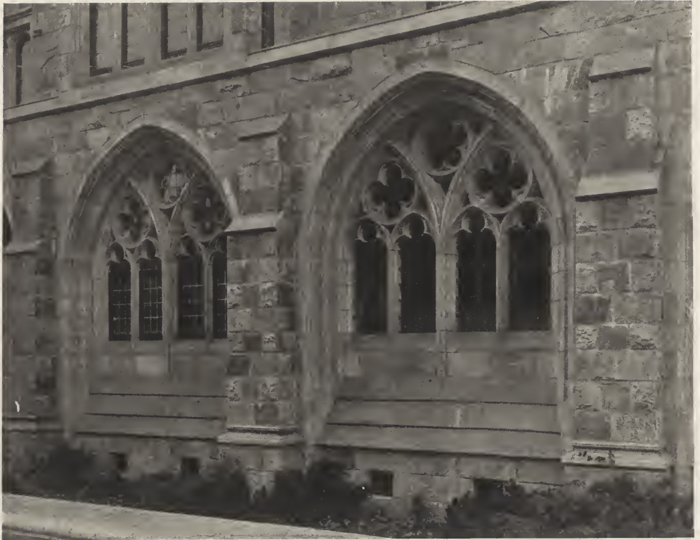
TRACERIED WINDOWS ABOVE MOAT-WALL IN ELM STREET— THE HARKNESS MEMORIAL QUADRANGLE AT YALE. James Gamble Rogers, Architect.
