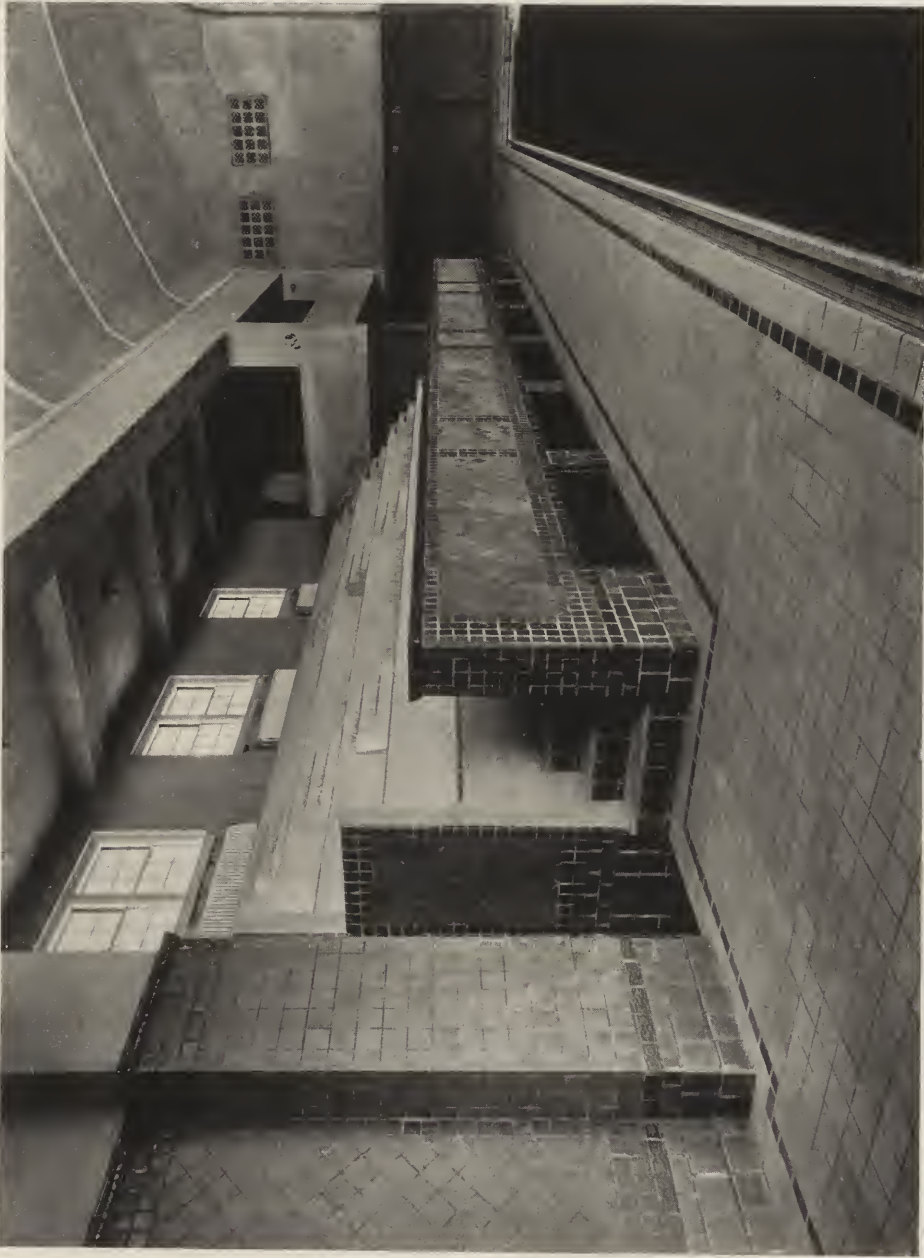
SPALDING SWIMMING POOL IN GYMNASIUM AT DART- MOUTH COLLEGE. RICH & MATHESIUS, ARCHITECTS.
