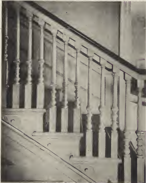
DETAIL OF STAIR BALUSTRADE, CLIVEDEN, GERMANTOWN (1763).
