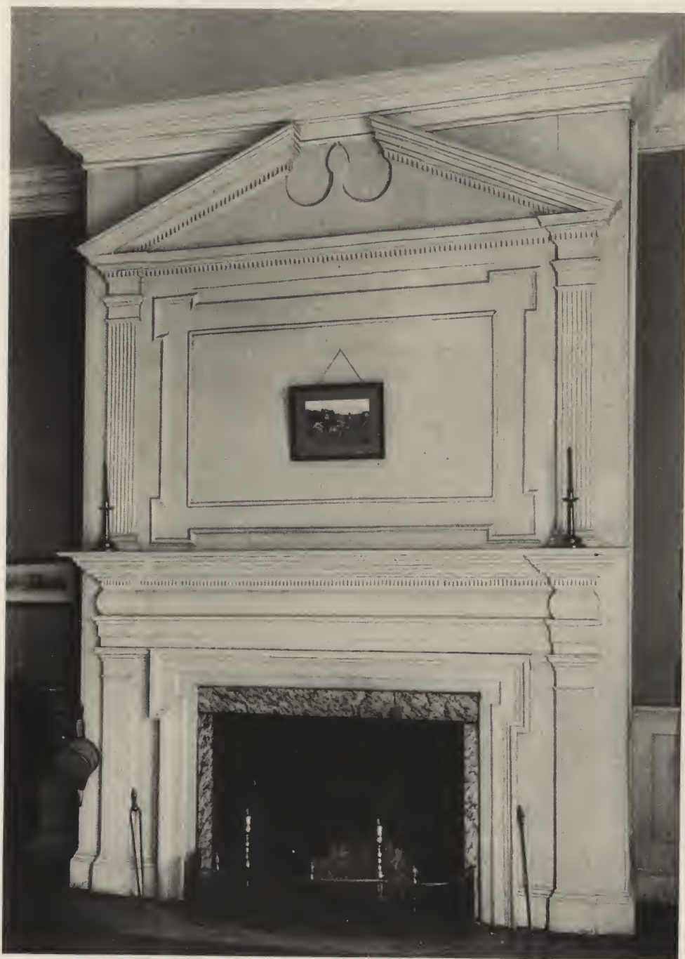
THE STATE BEDCHAMBER MANTELPIECE ON SECOND FLOOR OF EPHRAIM BLAINE HOUSE, CARLISLE, PA., 1792-97. EXAMPLE OF HIGH MANTEL WITHOUT ADJOINING WOODWORK.
