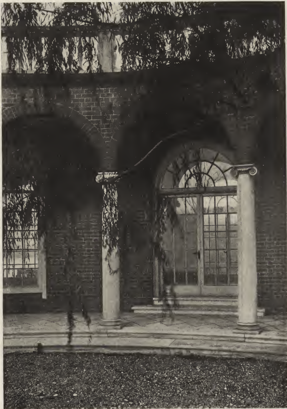
DETAIL OF CURVED PORCH—RESIDENCE OF LATHROP BROWN, ESQ., ST. JAMES, LONG ISLAND, N. Y. PEABODY, WILSON & BROWN, ARCHITECTS.
