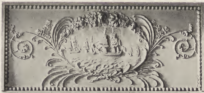
PANEL DETAIL, FRONT ROOM MANTEL, SECOND FLOOR, BELTZHOVER HOUSE, CARLISLE.
