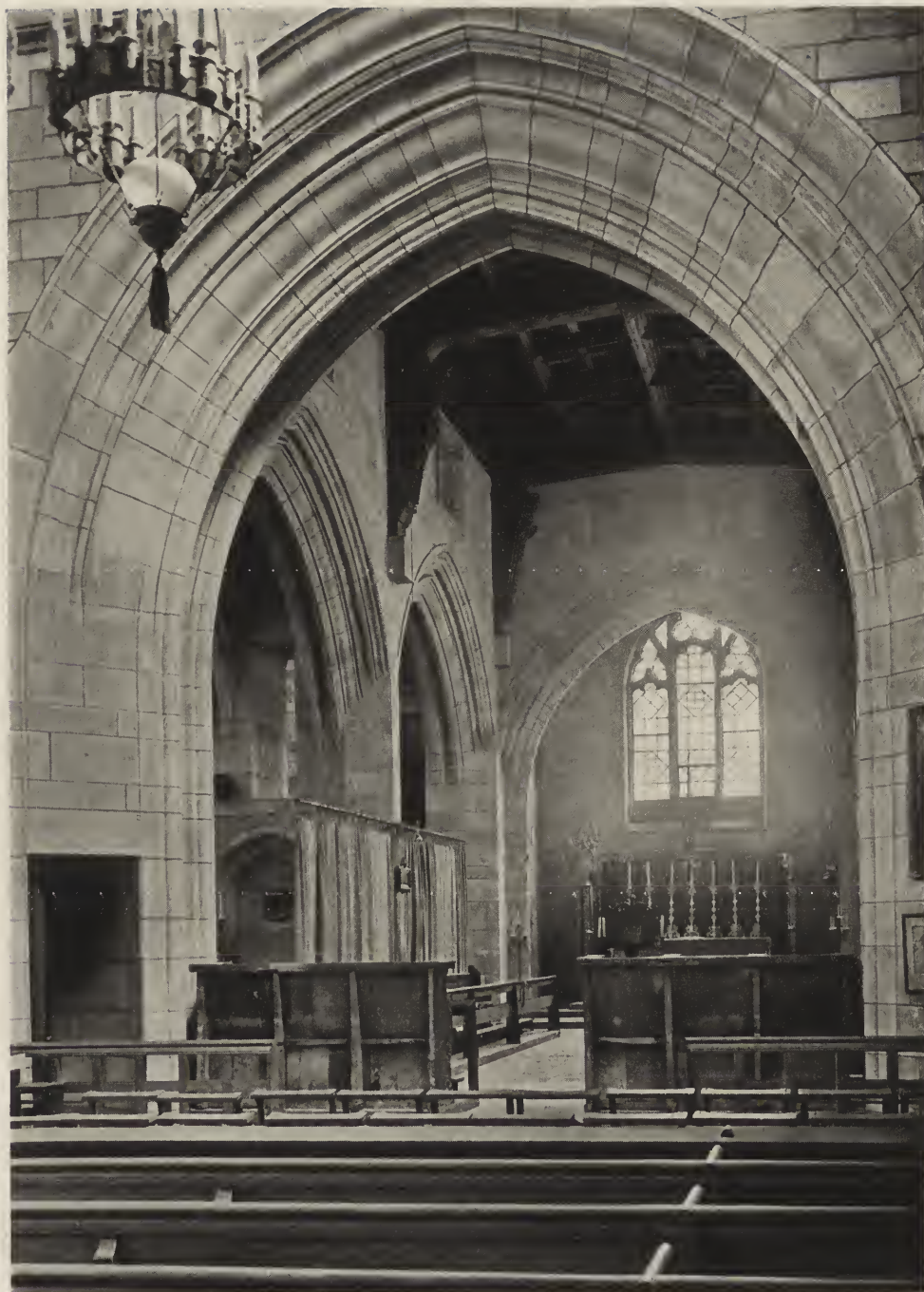
FRIARS' CHAPEL, CHURCH OF ST. VINCENT FERRER, NEW YORK CITY. BERTRAM G. GOODHUE, ARCHITECT.
