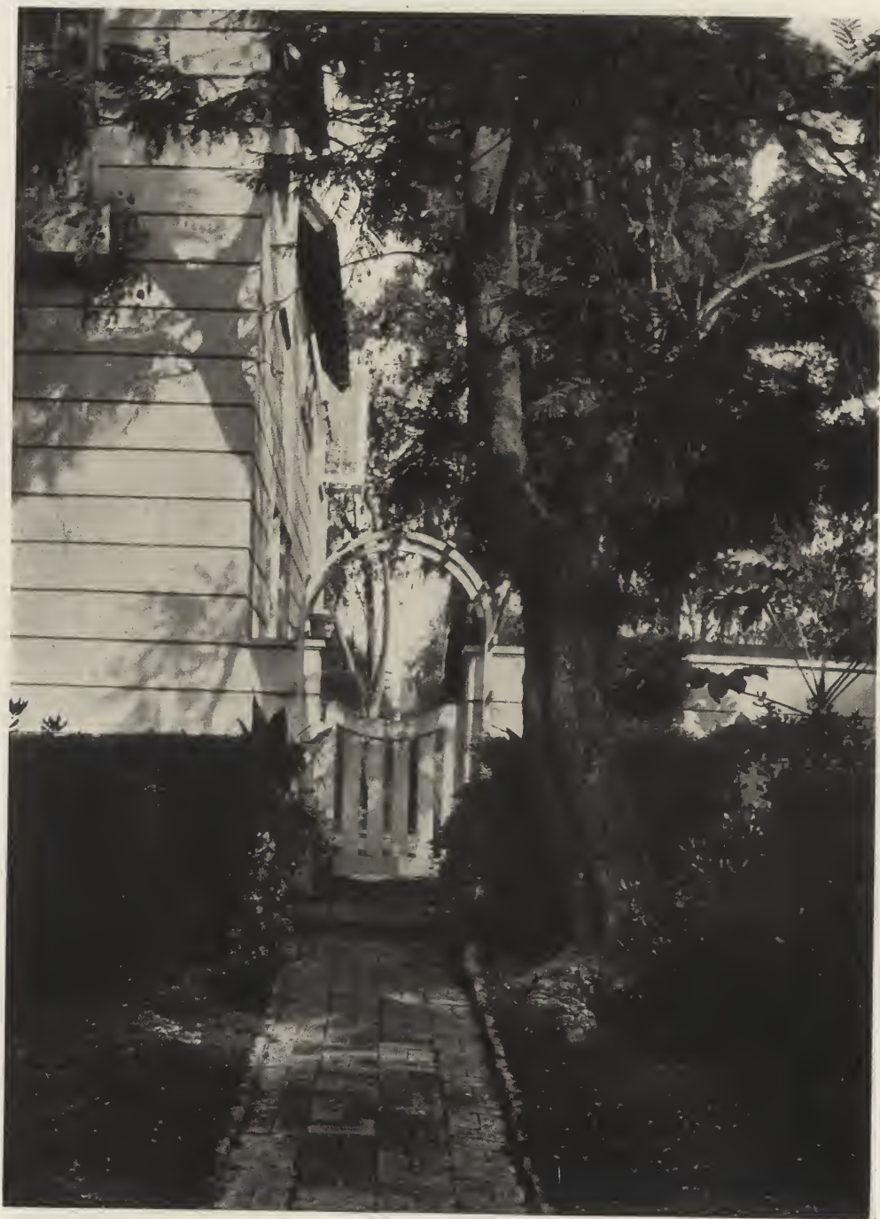
RESIDENCE OF MRS. GERTRUDE DAVIS, LOS ANGELES, CAL. PIERPONT & WALTER S. DAVIS, ARCHITECTS.
