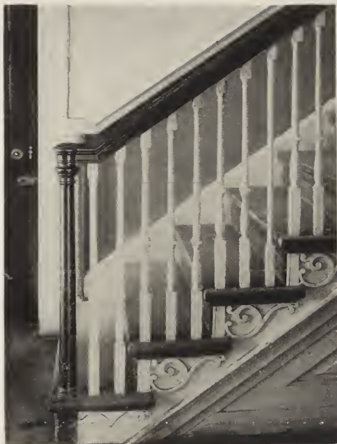
DETAIL OF STAIR BALUSTRADE, GOWEN HOUSE, MOUNT AIRY.
