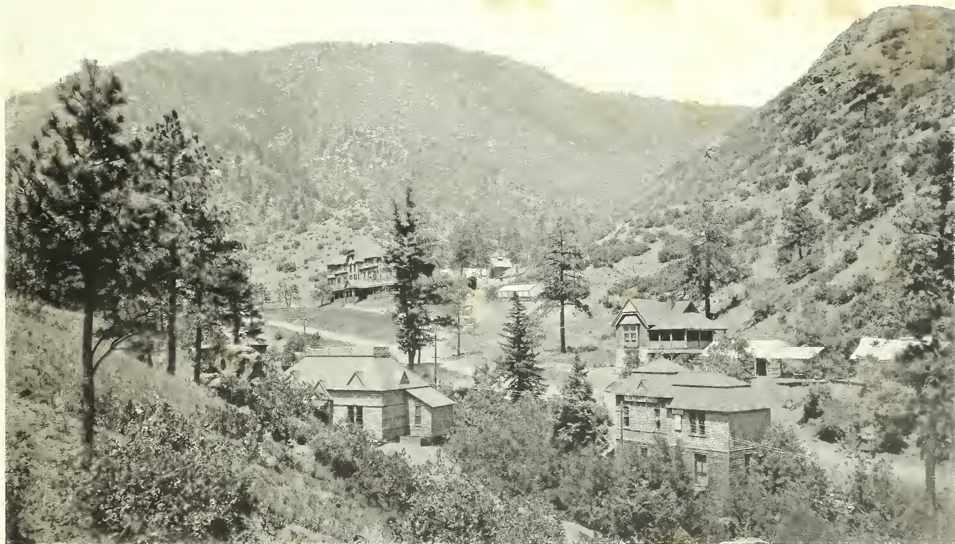
IRON SPRING COMPANY'S HOTEL AND PAVILIONS—MANITOU SPRINGS.
