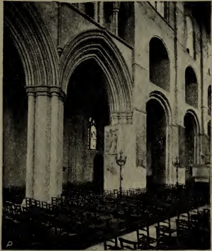
NAVE, NORTH SIDE.
