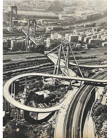
Construction of Viaduct Polcevera, Genoa, 1966. Http: // commons.wikimedia.org / wiki / file: construction _ Viaduct _ Polcevera _ 1966.jpg
