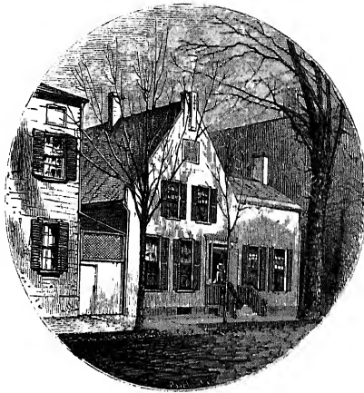
COLONIAL HOUSE, UNION STREET.
