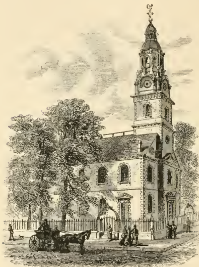
North Dutch Church. (On Fulton Street.)
