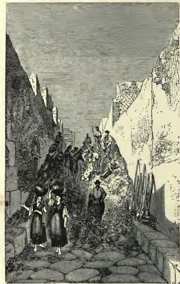
CLEARING A STREET.
