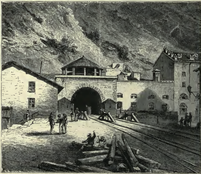
THE MONT CENIS TUNNEL, FROM THE ITALIAN SIDE.
