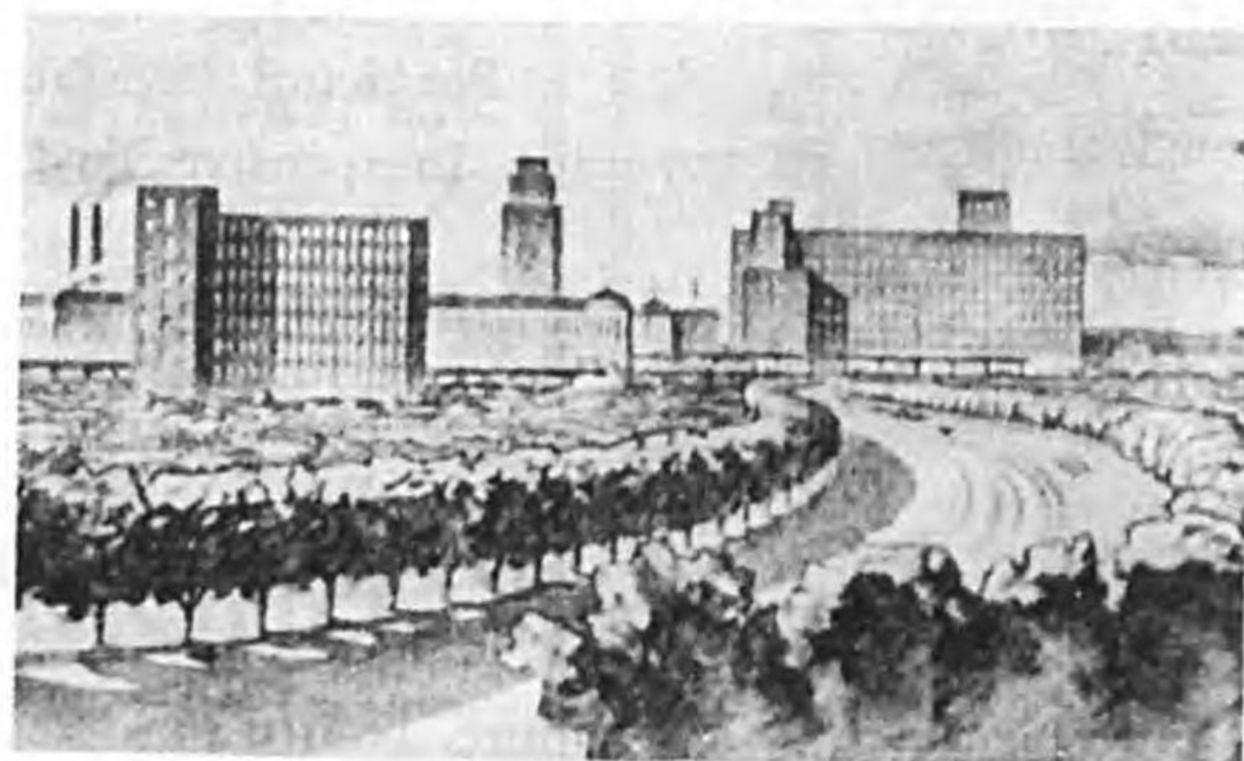
Siemens-Works at Berlin-Siemensstadt
