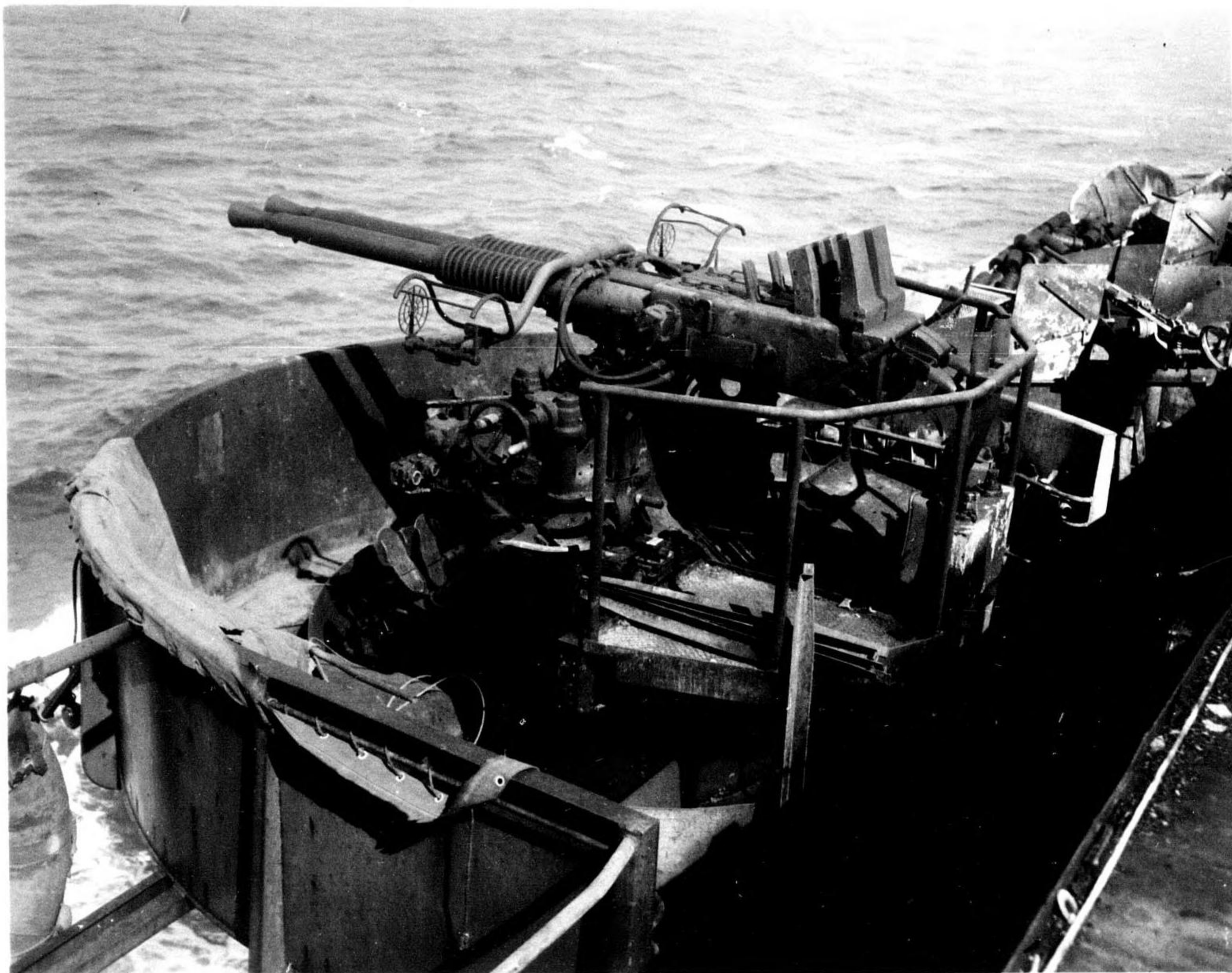
40 MM MOUNT DAMAGED BY BOMB, SHRAPNEL AND FIRE.
