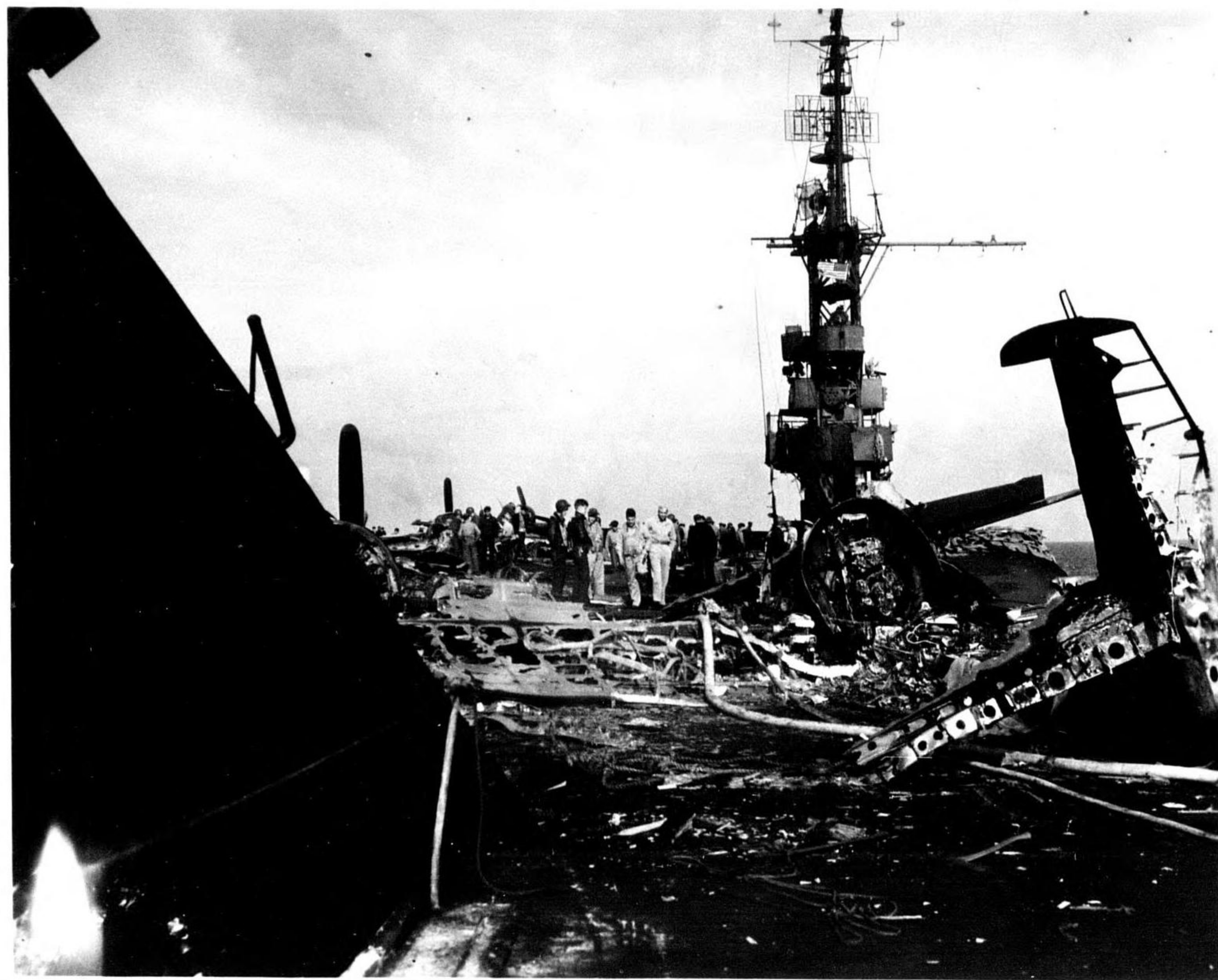
FLIGHT DECK LOOKING FORWARD FROM AFTER ELEVATOR.
