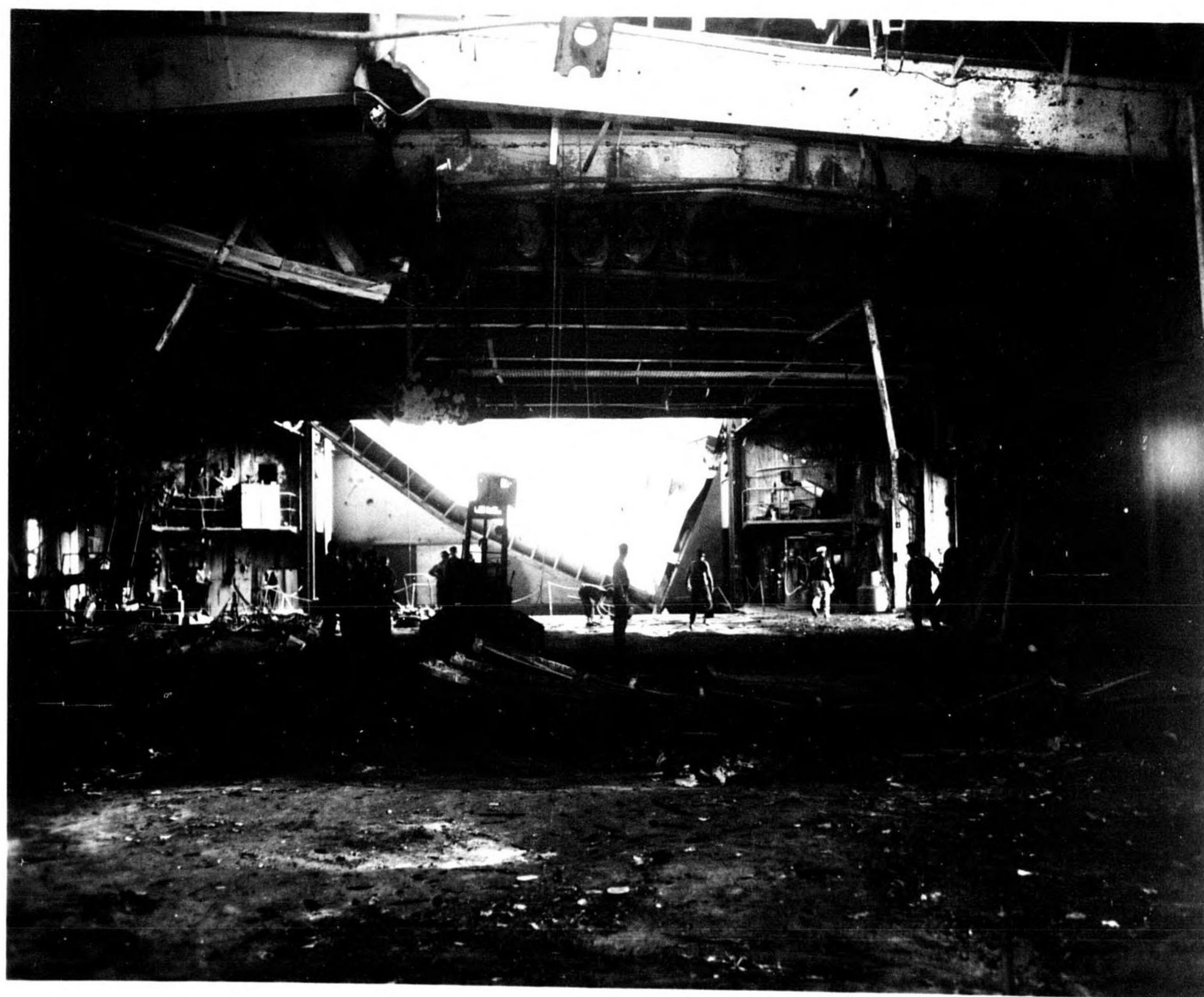
HANGAR DECK SPACE, AFTER CLEARING OF DEBRIS, SHOWING TILTED ELEVATOR AND GIRDER PENETRATED BY BOMB.
