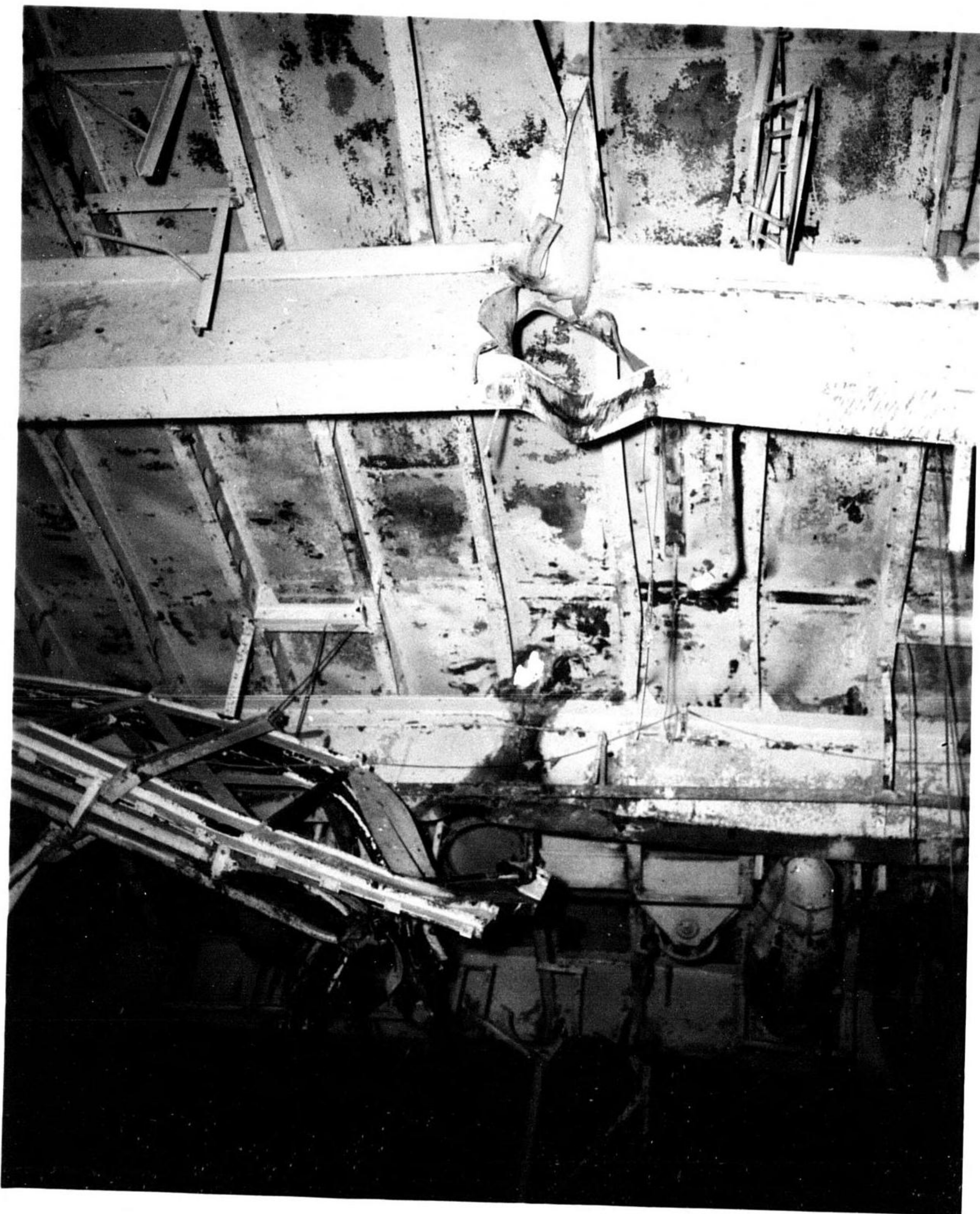
HANGAR SPACE OVERHEAD SHOWING THE HOLES WHERE BOMB PIERCED THE FLIGHT DECK AND SUPPORTING GIRDER.
