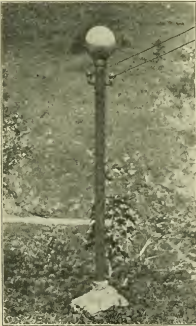
LIGHTING POST MADE FROM AN OLD BOILER TUBE, AND CASTING ADAPTING IT TO A STANDARD GLOBE.
