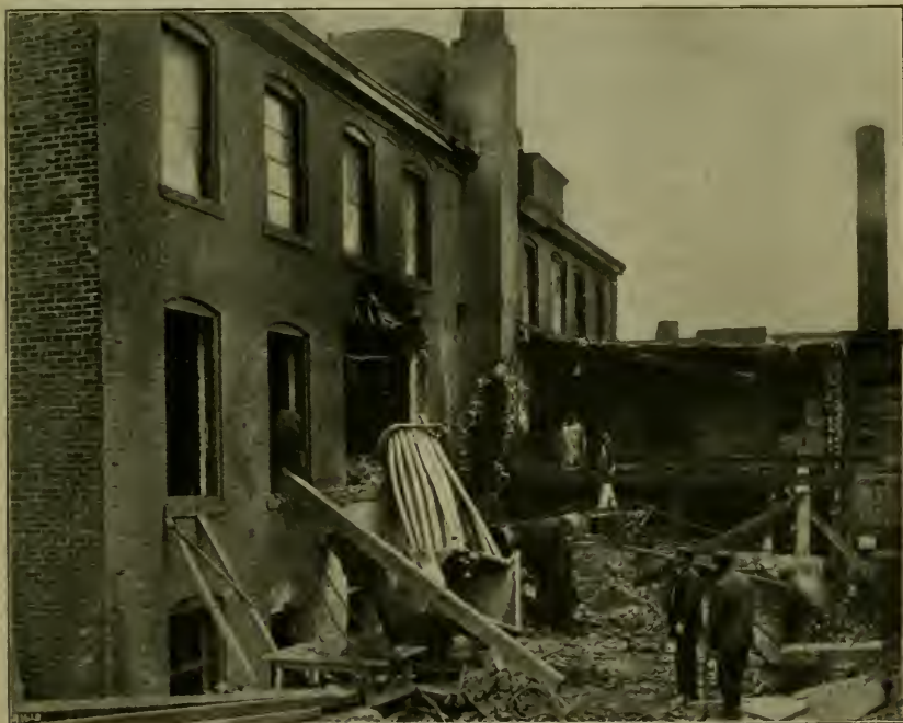
BOILER EXPLOSION AT BRIDGEPORT, CONN.
