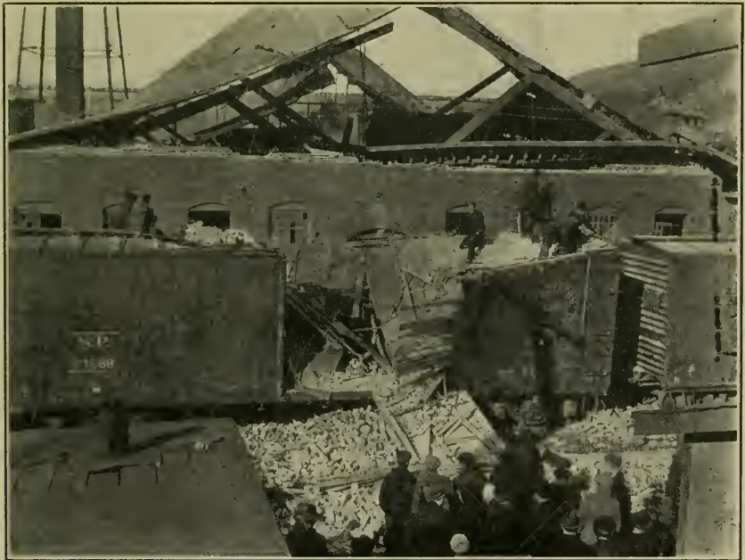
PAPER MACHINE DRYING CYLINDER EXPLOSION AT QUINCY, ILL.
