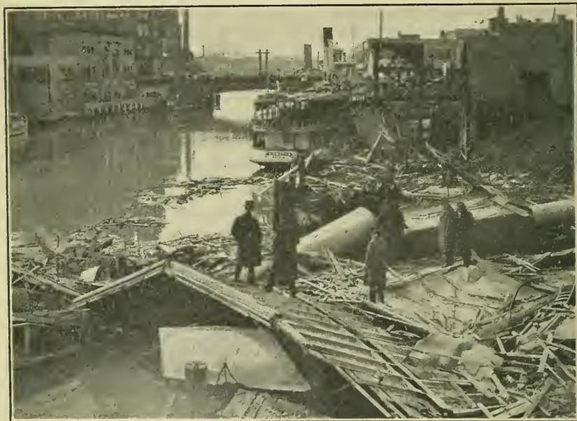
BOILER EXPLOSION AT PORT HURON, MICH.
