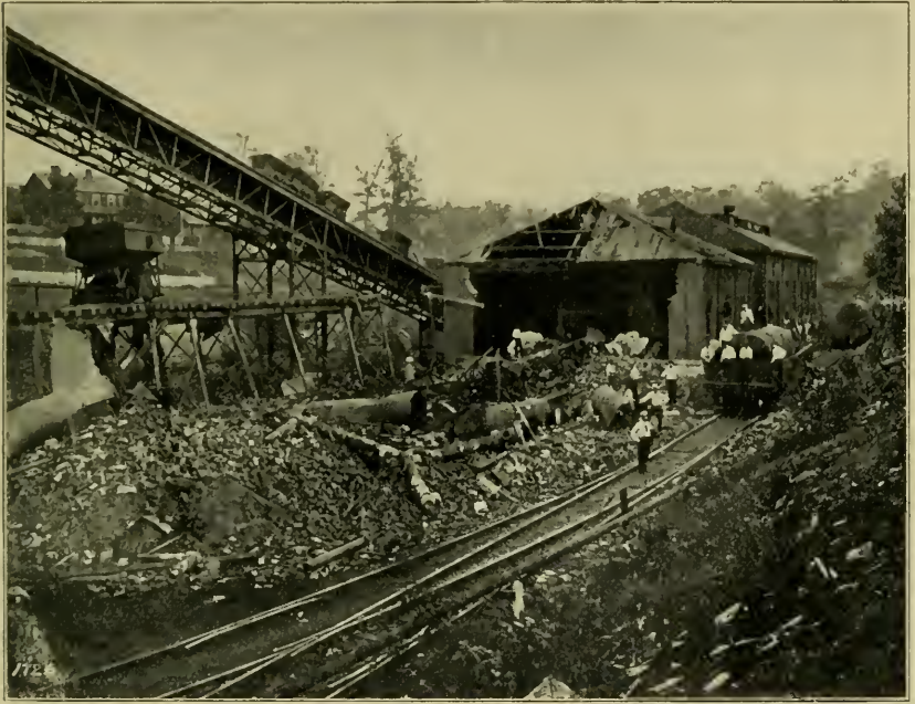
A SAFETY VALVE WHICH FAILED TO OPERATE CAUSED THIS EXPLOSION. ALL THAT REMAINED OF THE BOILER HOUSE WAS THE PILE OF WRECKAGE WHICH EXTENDS FROM THE LOWER LEFT HAND CORNER OF THE PICTURE TO THE BUILDING WHOSE ROOF WAS DAMAGED.
