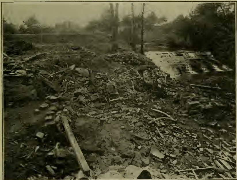
BOILER EXPLOSION IN A SAW MILL AT LeROY, OHIO.
