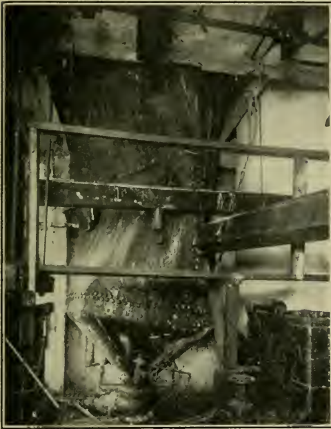
A COLLAPSED COOKING TANK.
