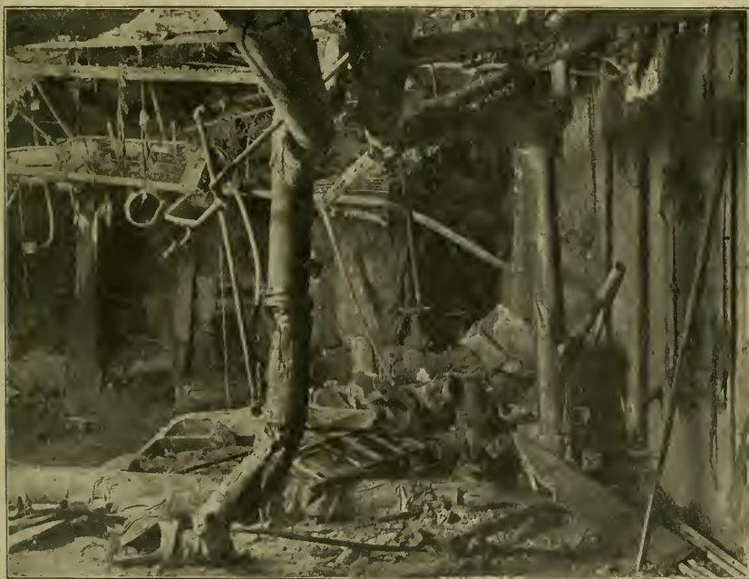
HEATING BOILER EXPLOSION AT ST. LOUIS.
