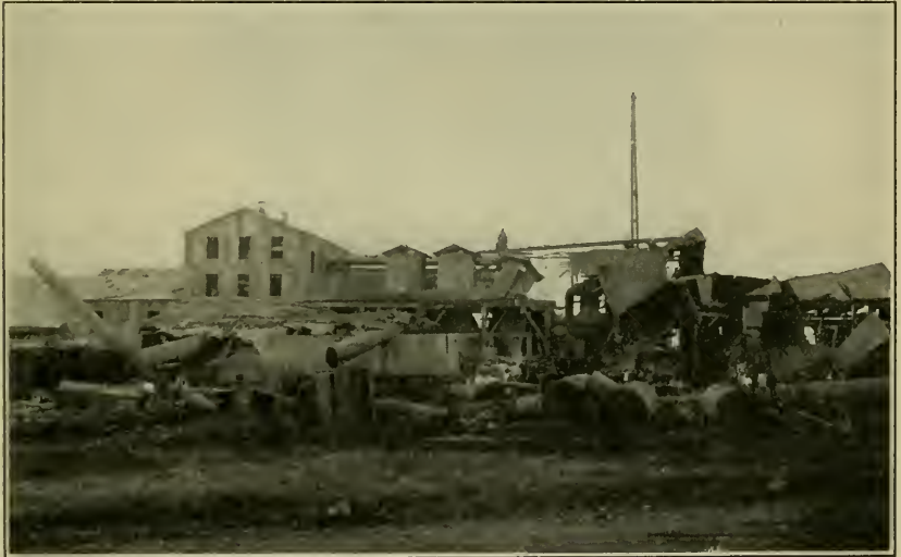
BOILER EXPLOSION AT LOREAUVILLE, LA.
