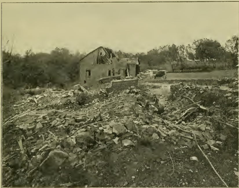
UNFAMILIARITY WITH THE PROPER ADJUSTMENT OF SAFETY VALVES CAUSED THIS BOILER EXPLOSION.
