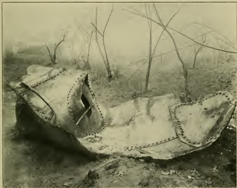
BOILER EXPLOSION CAUSED BY CORROSION.
