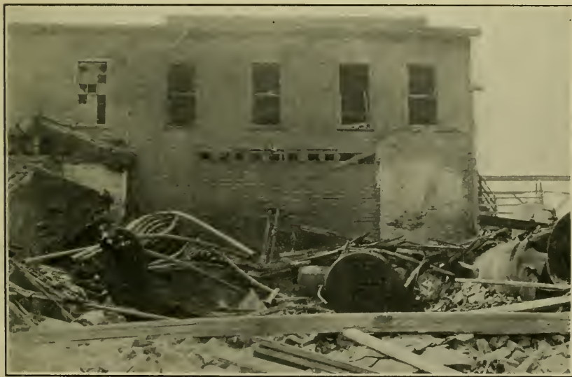
BOILER EXPLOSION AT A LOUISIANA COTTON OIL MILL.
