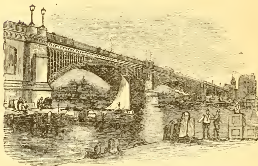
CHESTNUT STREET BRIDGE.
