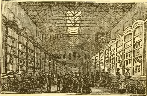
FARMERS' MARKET HOUSE. INTERIOR VIEW.
