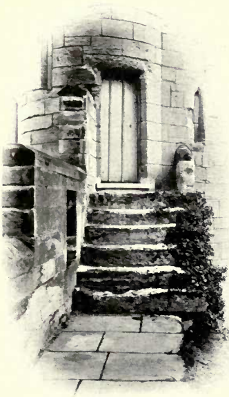
BATTELEMENT STEPS, WARWICK CASTLE.
