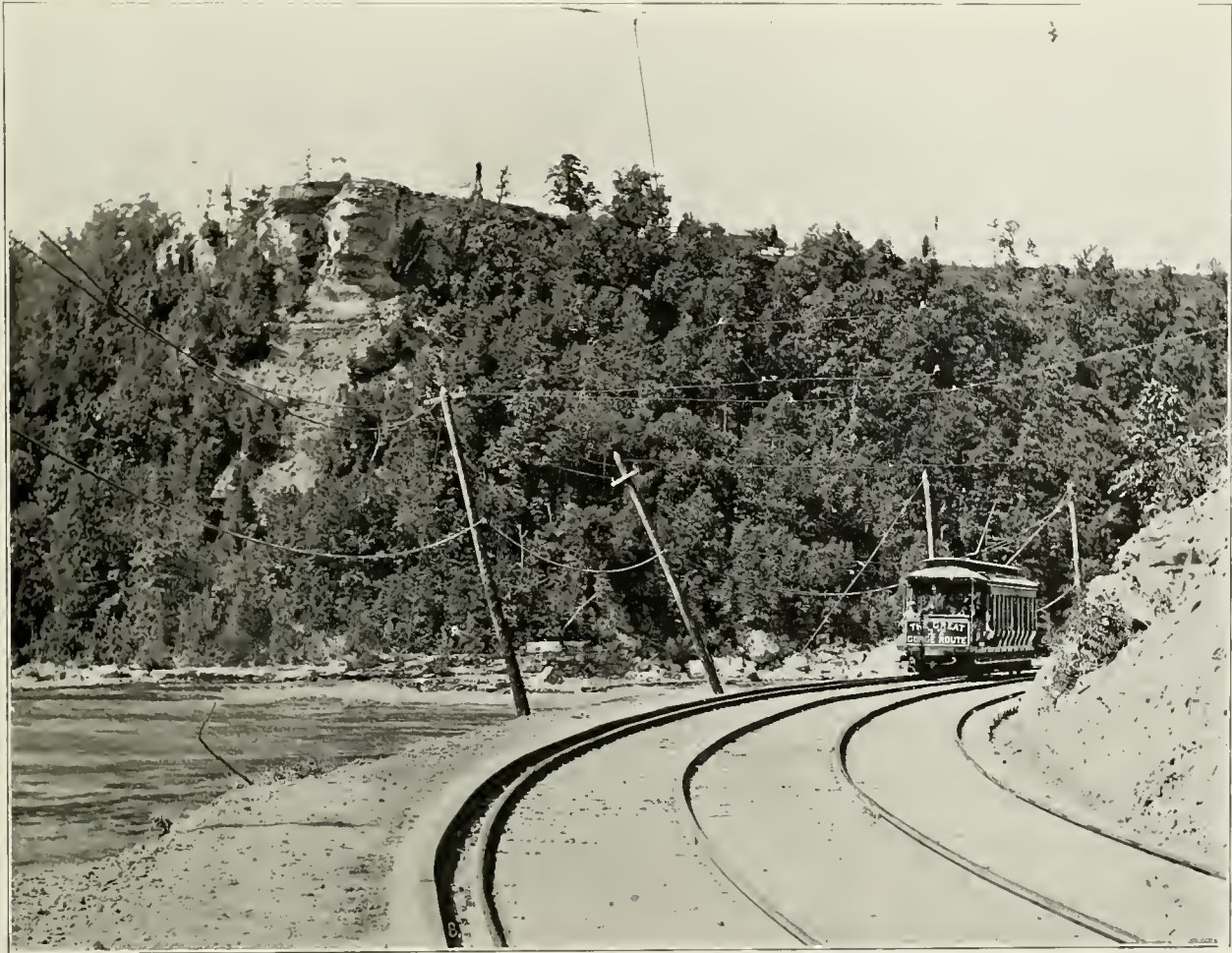
THE LOWER END OF THE GORGE RAILROAD.
