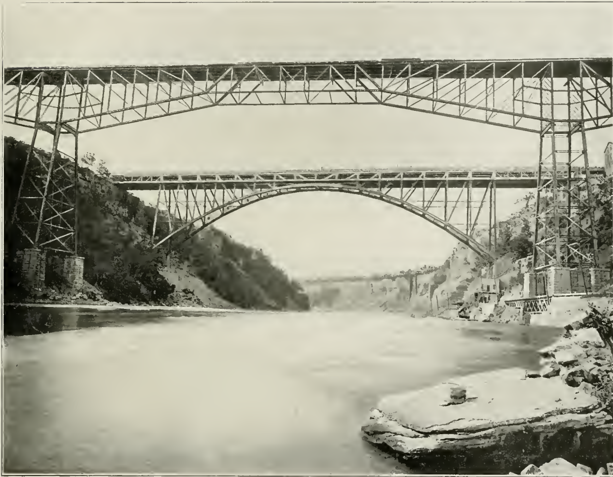
THE BRIDGES ACROSS THE GORGE AT SUSPENSION BRIDGE
