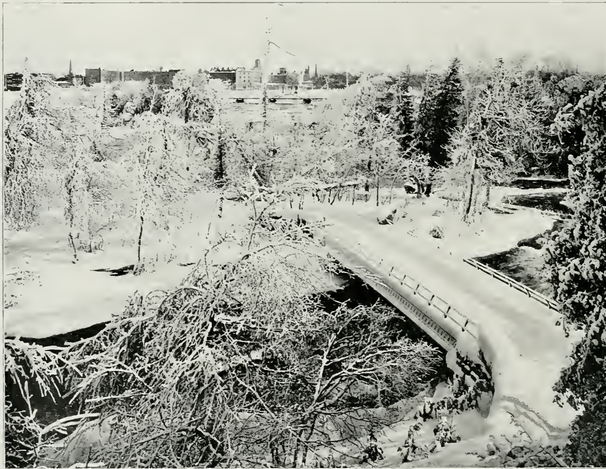
THE BRIDGE TO LUNA ISLAND IN WINTER
