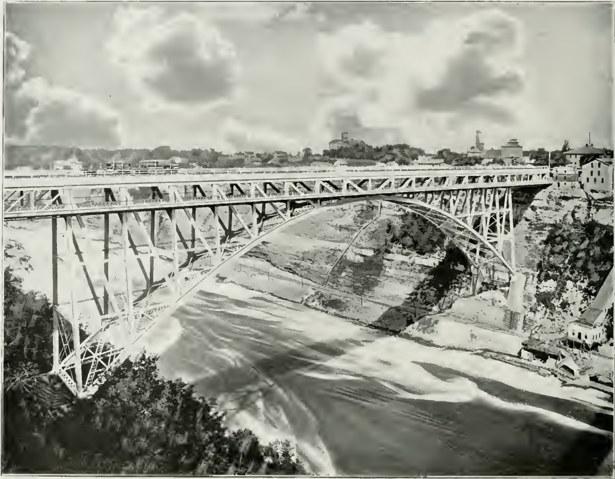
GRAND TRUNK RAILWAY STEEL ARCH BRIDGE
