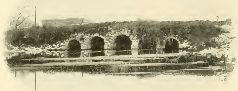
AGASSIZ BRIDGE IN THE FENS
