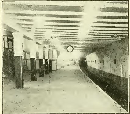
MILK STATION, WASHINGTON STREET TUNNEL
