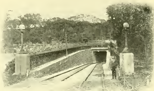
ENTRANCE TO SUBWAY, PUBLIC GARDEN
