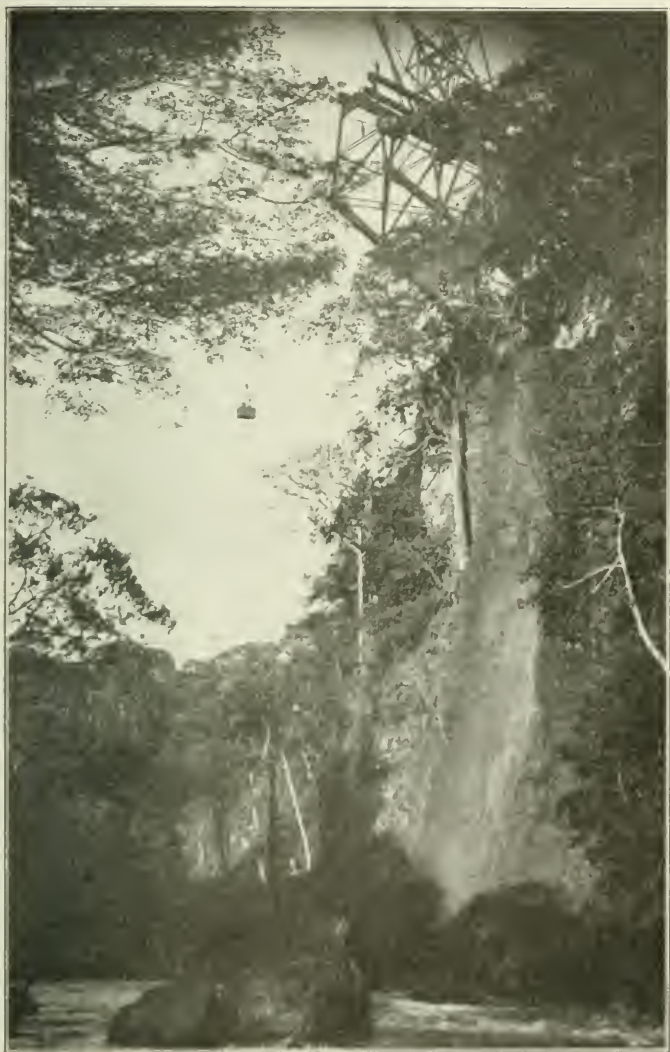
RIO GRANDE BRIDGE DURING CONSTRUCTION
