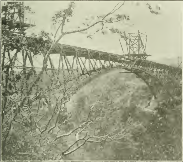
RIO GRANDE BRIDGE NEARING COMPLETION
