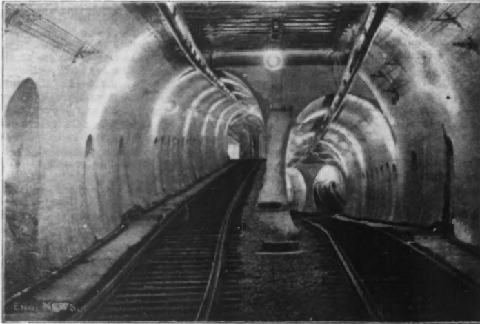
FIG. 1.—BELLMOUTHS UNDER TREMONT ST. NEAR HOLLIS ST., SHOWING PASSAGE OF SOUTH BOUND SHAWMUT AVE. TRACK UNDER NORTH BOUND TREMONT ST. TRACK.
