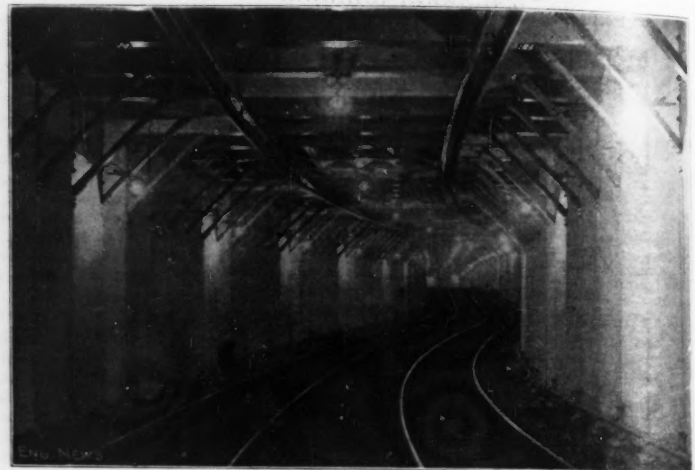
FIG. 2.—TWO-TRACK SUBWAY UNDER BOYLSTON ST. MALL, BOSTON COMMON, LOOKING EAST.
