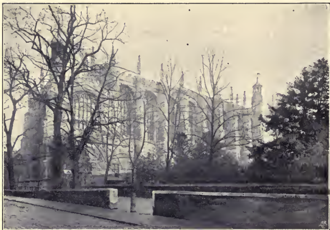
THE CHAPEL, FROM THE SOUTH-WEST.
