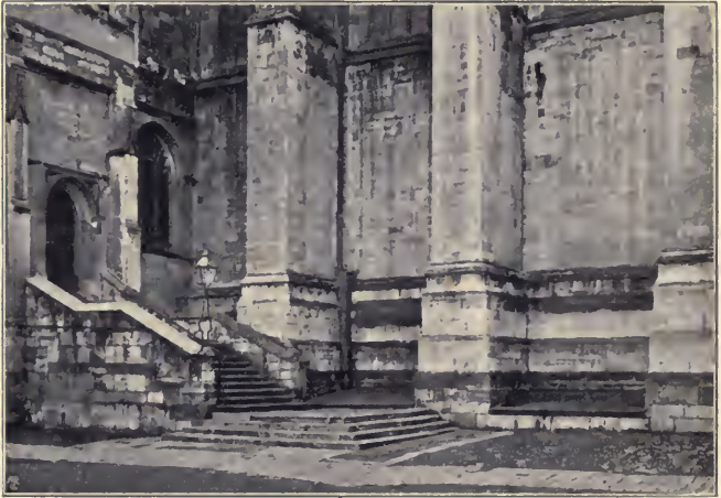
NORTH SIDE OF THE CHAPEL, SHOWING THE STEPS WHERE ABSENCE IS CALLED, AND THE ORIGINAL FIVES COURT.
