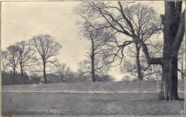
THE WALL AND BAD CALX.
