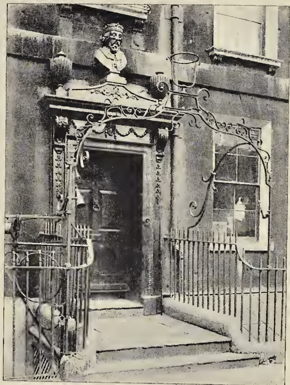
DOORWAY IN ALFRED STREET.
