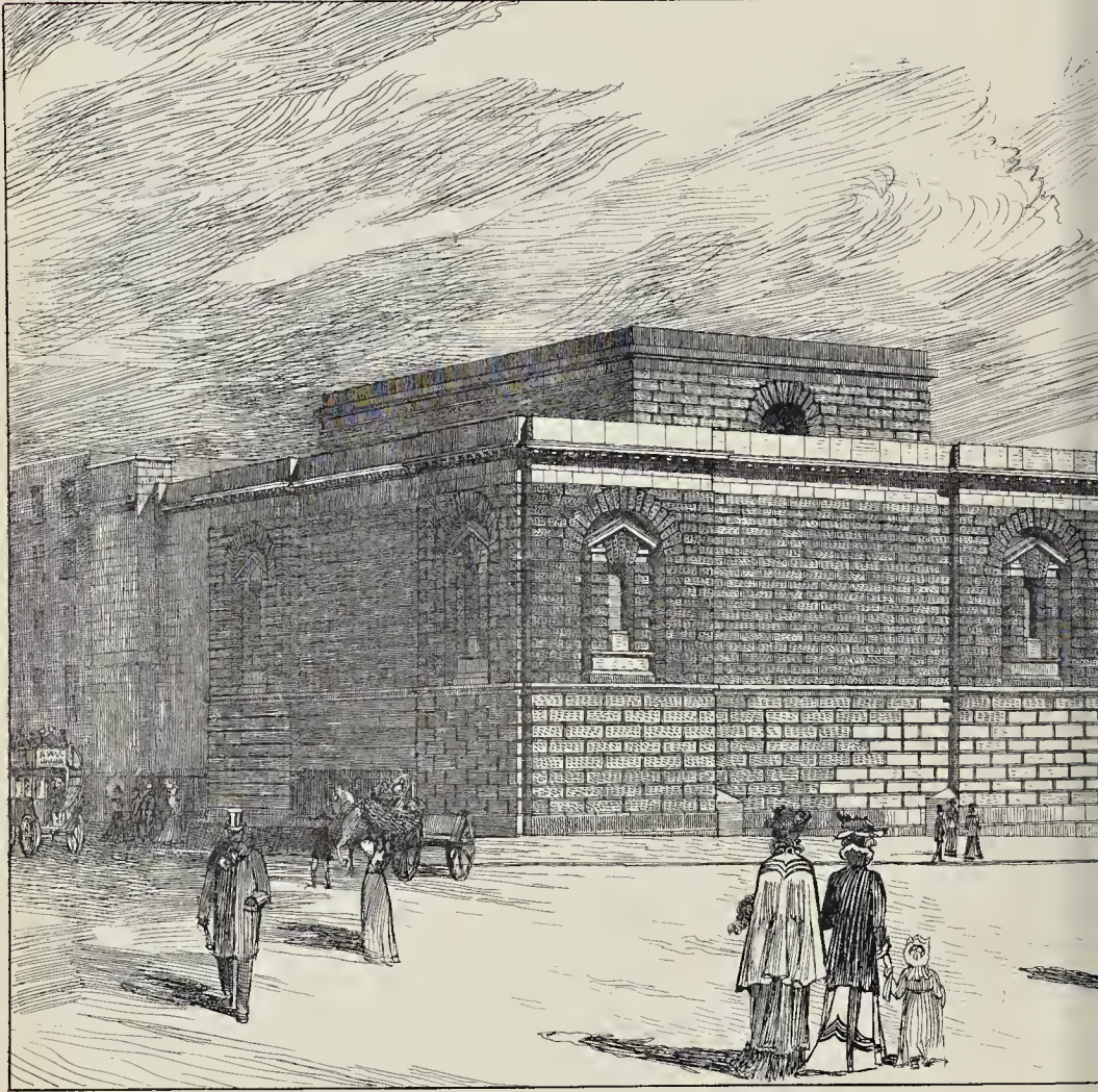
NEWGATE PRISON SHORTLY TO BE DEMOLISHED. BUILDING FROM A DRAWING BY
