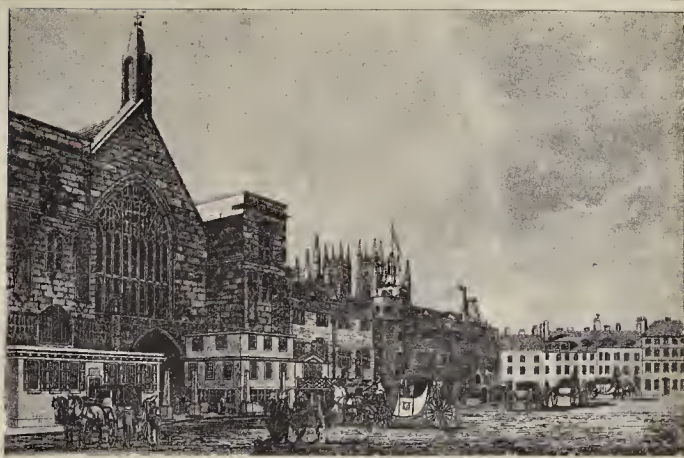
NEW PALACE YARD.
