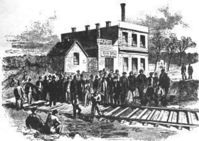
DRIVING THE FIRST SPIKE ON THE ATCHISON AND PIKE'S PEAK RAILROAD.—[SKETCHED BY WILLIAM M. MERRICK.]
