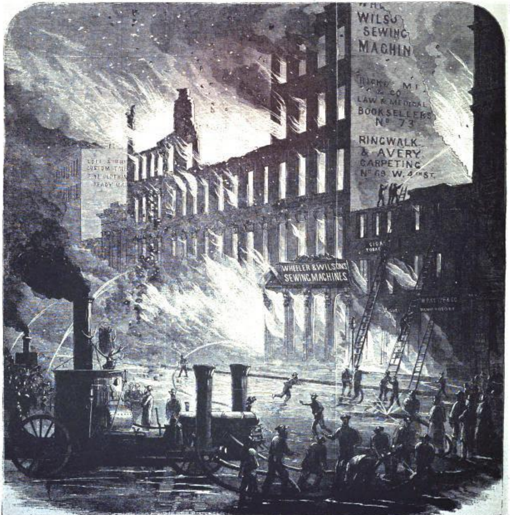
THE GREAT FIRE IN CINCINNATI, MARCH 24, 1866—BURNING OF PIKE'S OPERA-HOUSE.—SKETCHED BY A. R. WADE.—[SEE FIRST PAGE.]
