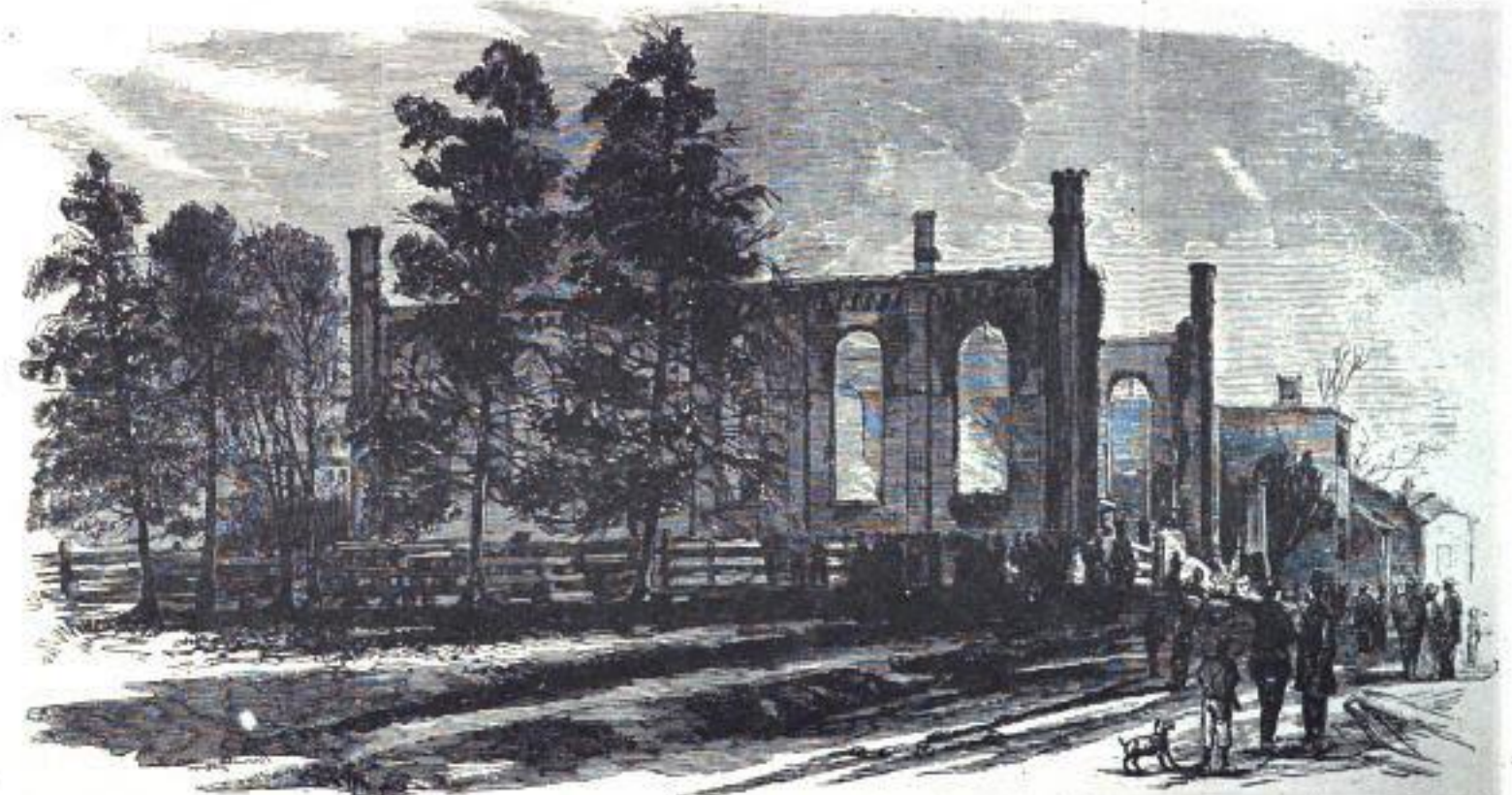
FIRES AT PETERSBURG, VIRGINIA—RUINS OF THE COLORED BAPTIST CHURCH ON HARRISON STREET.—[PHOTOGRAPHED BY LAZELLE & M-MOLLEN, PETERSBURG, VA.]
