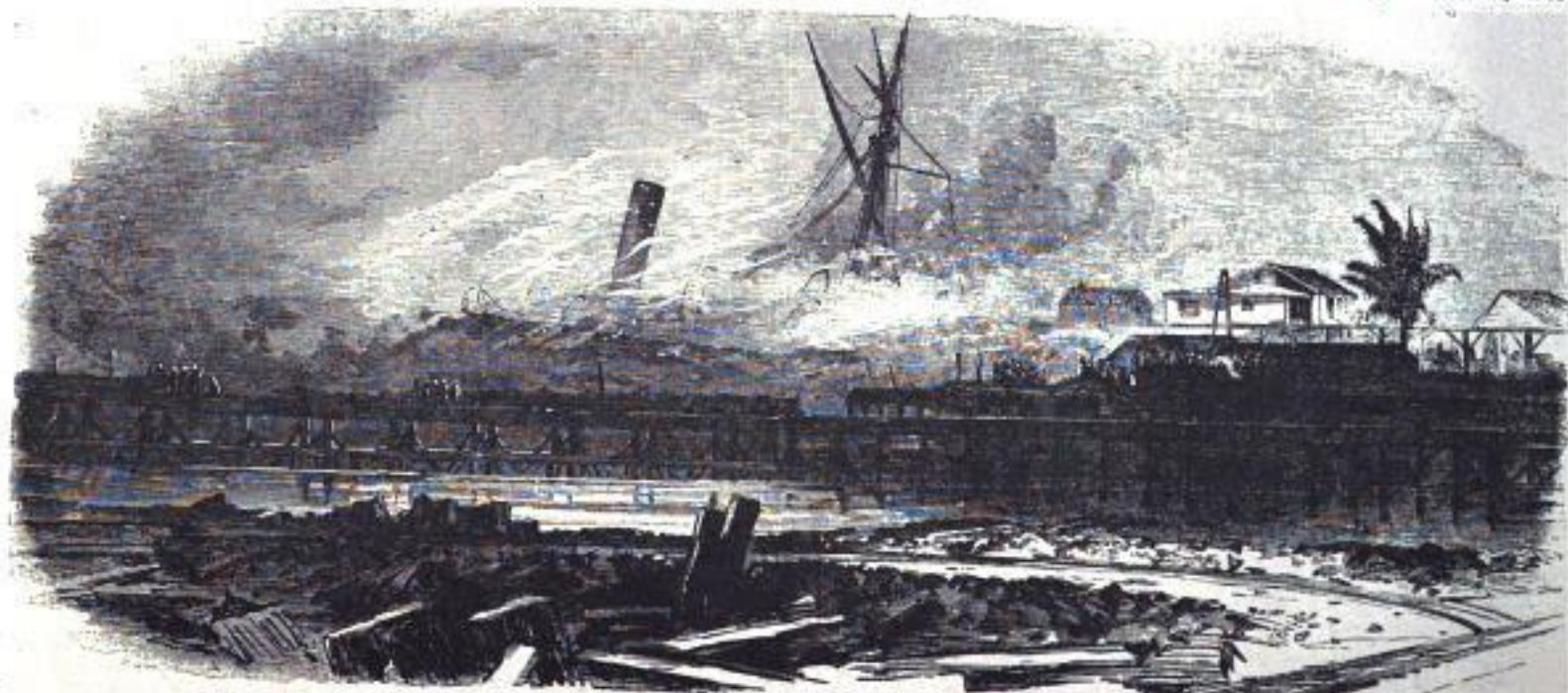
EXPLOSION AT ASPINWALL.—THE WHARF AND THE "EUROPEAN" ON FIRE.—(PHOTOGRAPHED IMMEDIATELY AFTER THE EXPLOSION BY J. MARTINEZ, ASPINWALL.)
