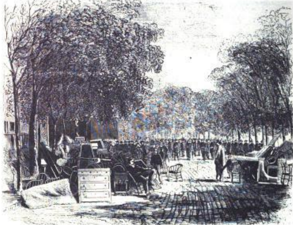
THE FIRE IN SARATOGA—BROADWAY THE MORNING AFTER THE FIRE.—[PHOTOGRAPHED BY A. S. AVERY.]
