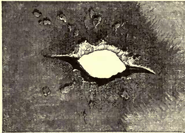
Sheet-lead punctured by lightning.
