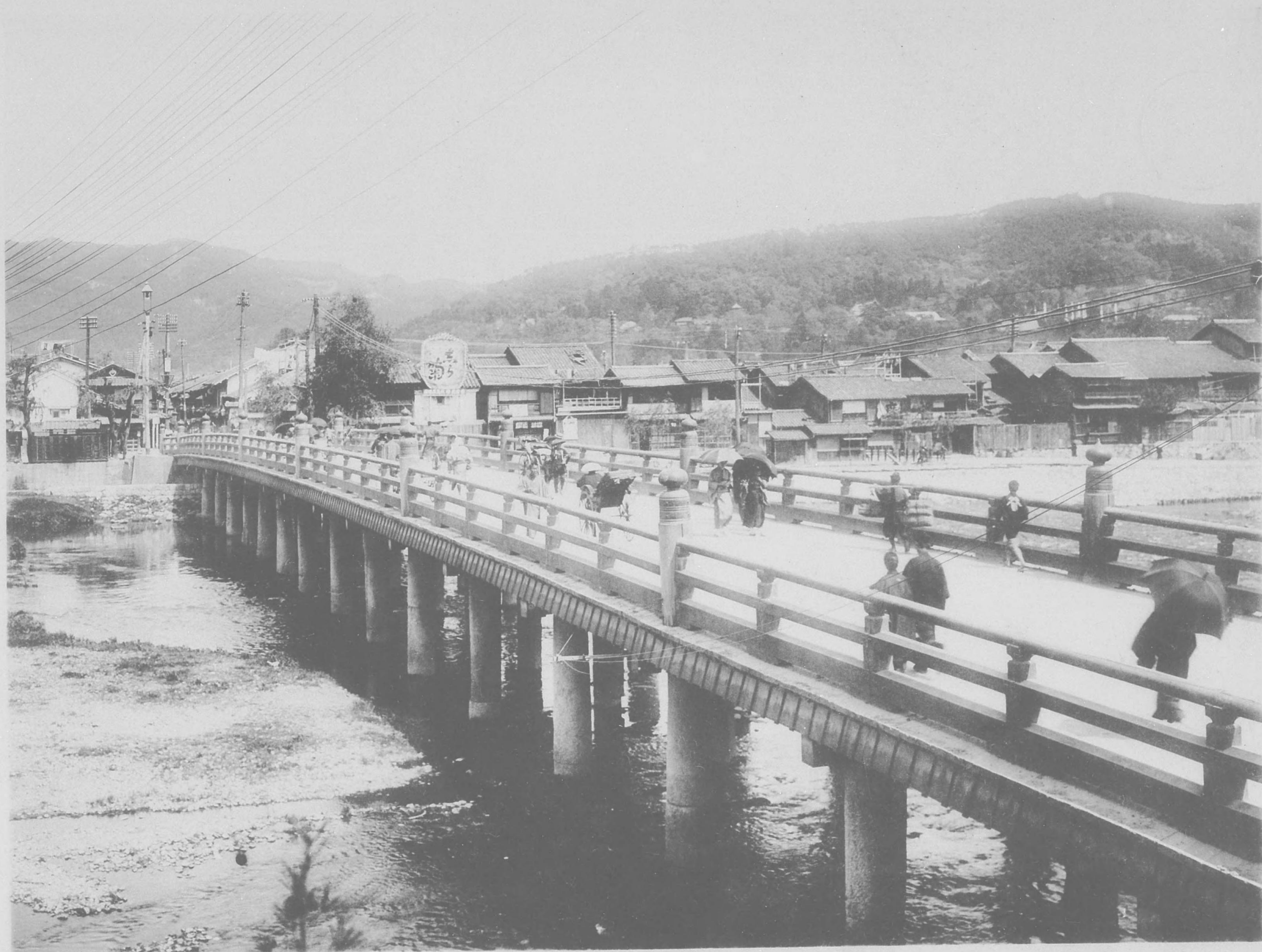
A large wooden bridge over the Kamogawa, on Sanjō-dōri; purely Japanese in style and supported on huge granite pillars.
