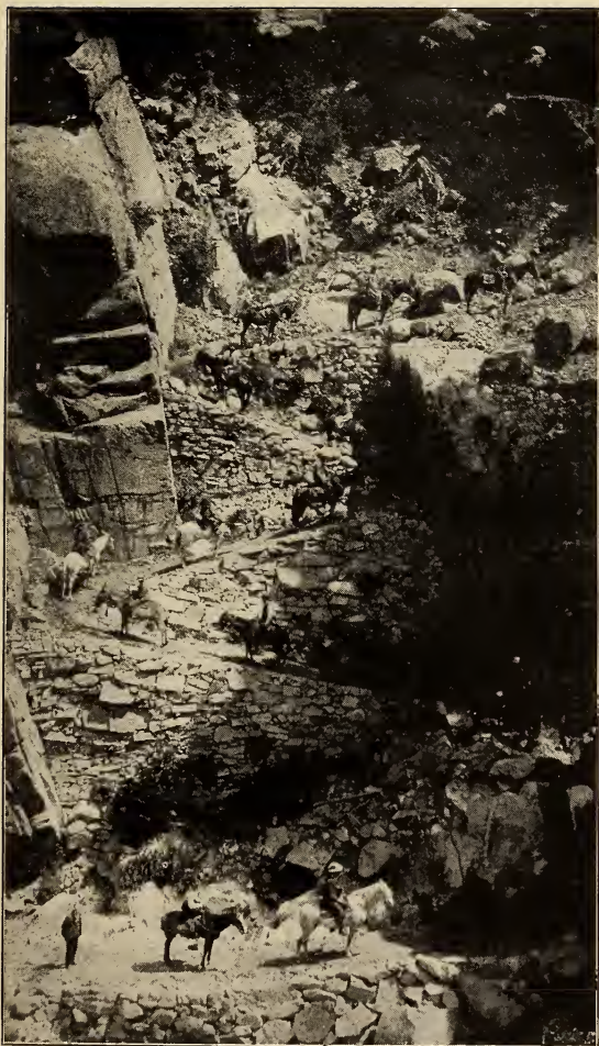
STAIRWAY ON CLOUD'S REST TRAIL.
