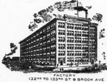
FACTORY 132 ND TO 133 RD ST & BROOK AVE
