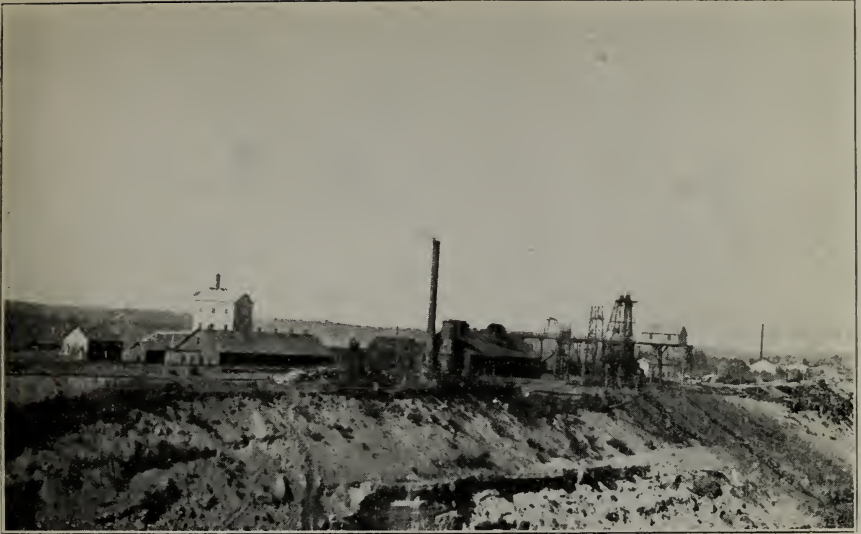
A. HEAD-FRAME, CONCENTRATING PLANT, AND PART OF OPEN PIT AT THOMPSON MINE, NEAR CROSBY. LOOKING NORTHEASTWARD PHOTO BY CARL ZAPFFE
