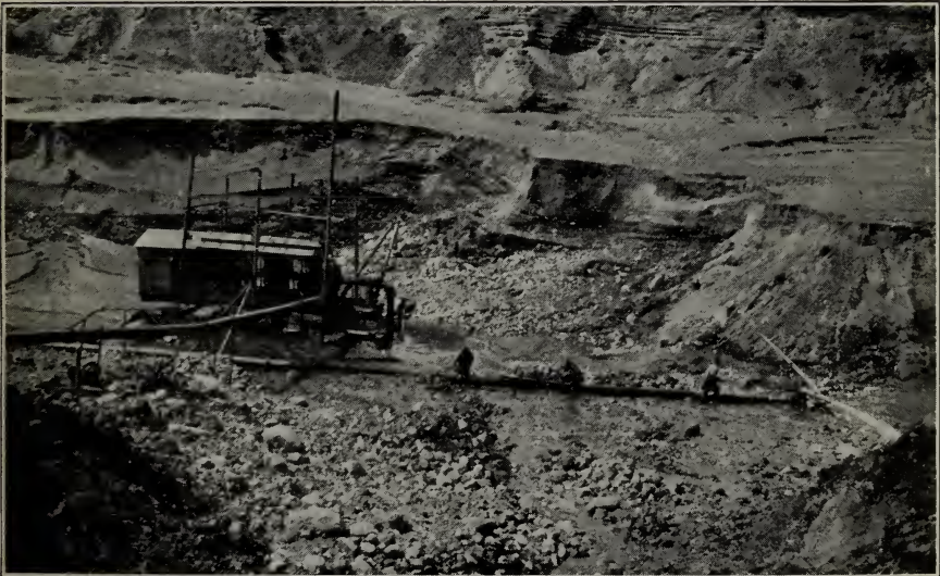
B. REMOVING OVERBURDEN BY HYDRAULIC METHOD AT THE HILLCREST MINE, NEAR IRONTON. SHOWS GIANT NOZZLE, CENTRIFUGAL PUMP, AND DISCHARGE PIPE PHOTO BY CARL ZAPFFE
