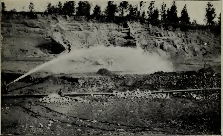
A. REMOVING OVERBURDEN BY HYDRAULIC METHOD AT THE ROWE MINE, NEAR RIVERTON. SHOWS STREAM OF WATER ISSUING FROM GIANT NOZZLE WASHING DOWN SAND AND CLAY
