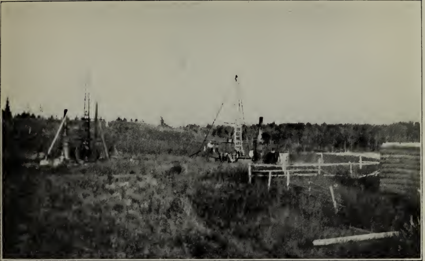
A. EXPLORATION BY DRILLING IN THE CUYUNA DISTRICT
