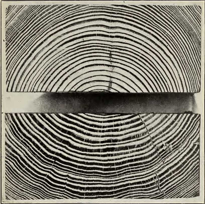
CROSS-SECTION OF TWO LOBLOLLY PINE BEAMS WITH APPROXIMATELY EQUAL RATES OF GROWTH, BUT WITH DIFFERENT PROPORTIONS OF SUMMER WOOD.
