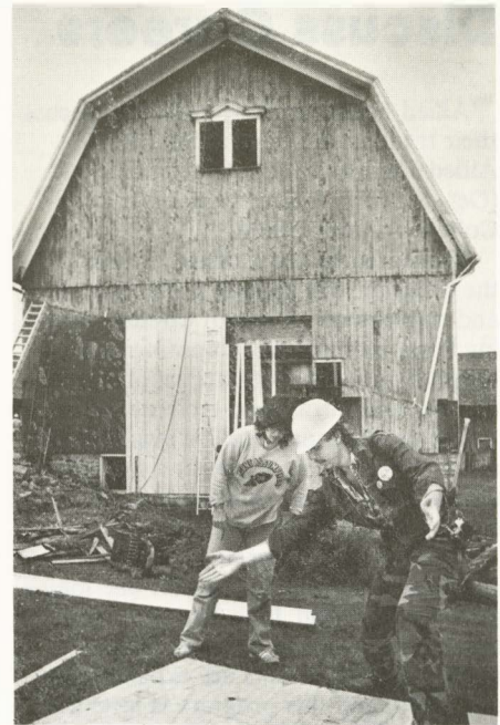
Restoration under way last Saturday morning at the Red Barn
