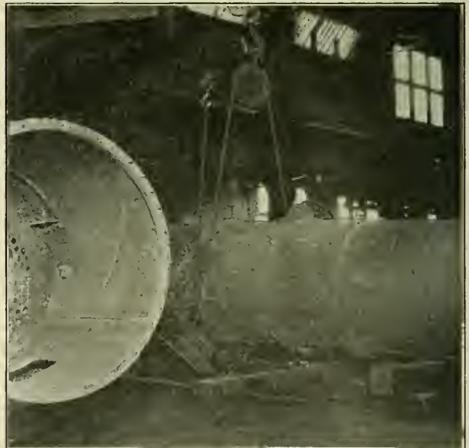
Fig. 8—Fixture Used in Rolling Boilers
