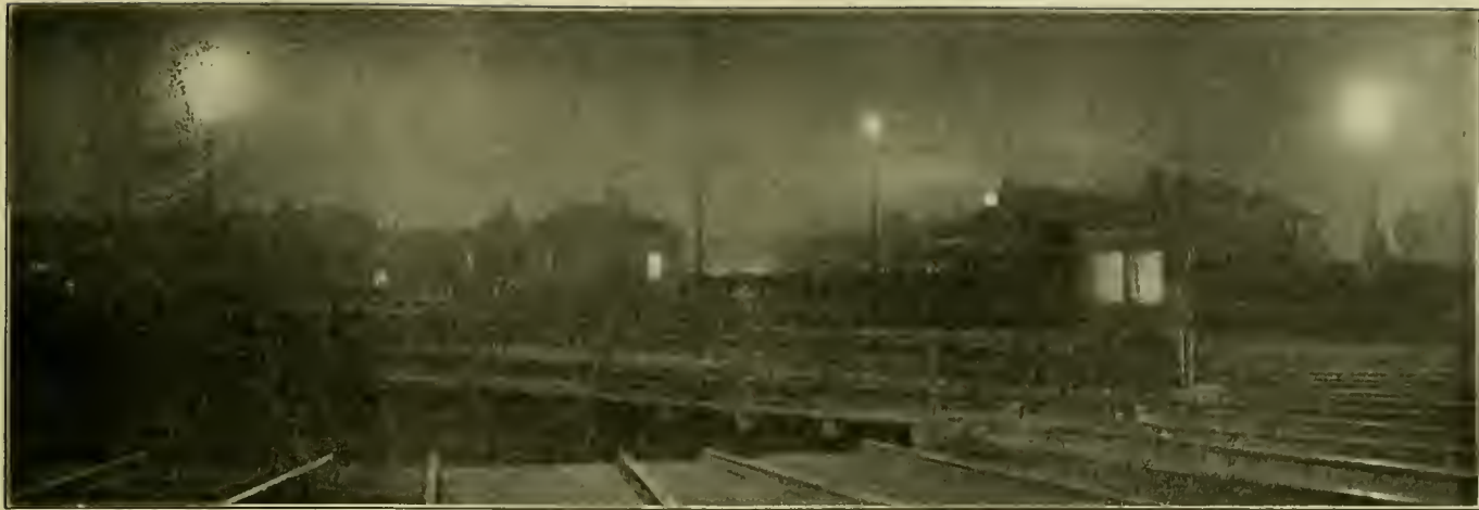
Floodlighting for the Turntable and Lead Tracks. Photograph by the American Lighting Company, Chicago
