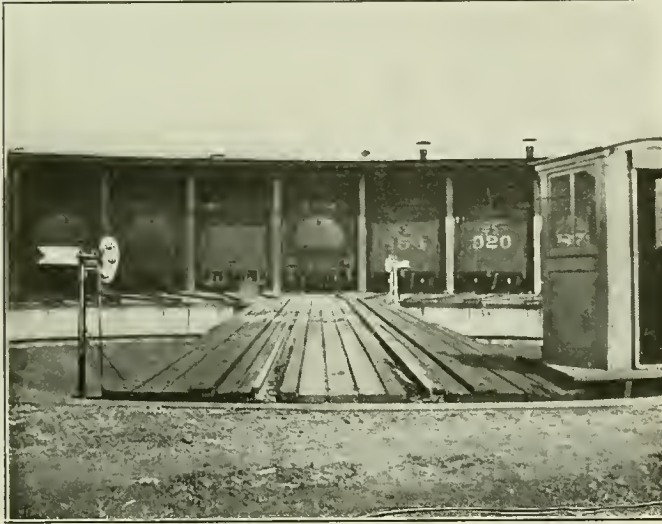
Fig. 1—View Showing Indicator Applied at Each End of the Turntable
