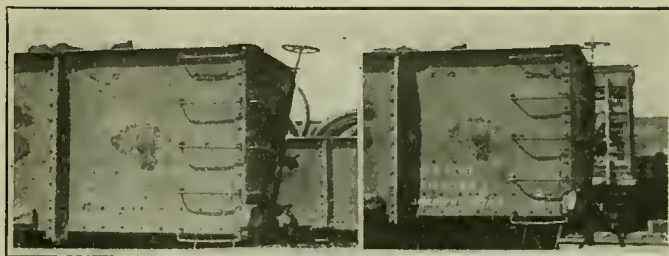
A Bulged End Repaired by Two Men in 20 Minutes
