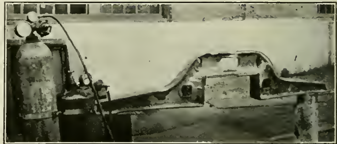
Fig. 6.—Needle Beam, Shown in Fig. 5, As Repaired by Gas Welding
