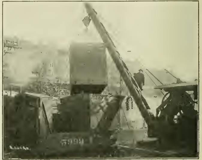
Locomotive Crane Placing a Loaded Container on the Car
