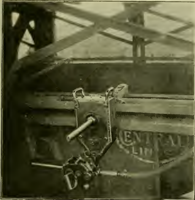
Fig. 6—Power Jack In Position to Straighten the Side of a Hopper Car
