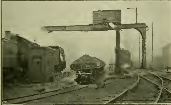
Water Pit with Overhead Crane and Side Dump Cars Used for Handling Ashes
