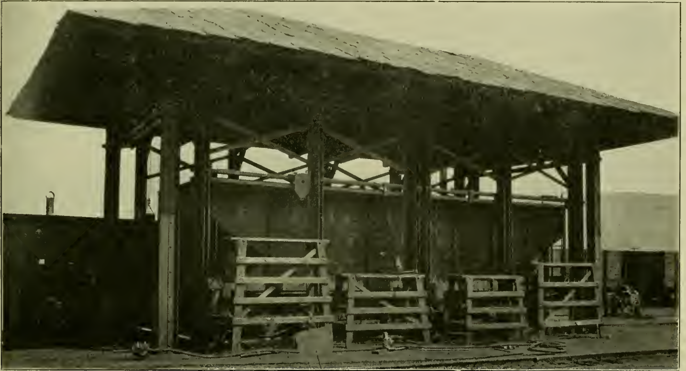
Fig. 1—Jacking Stall at Avis Shops, Showing Jacking Bars and Power Operated Jack
