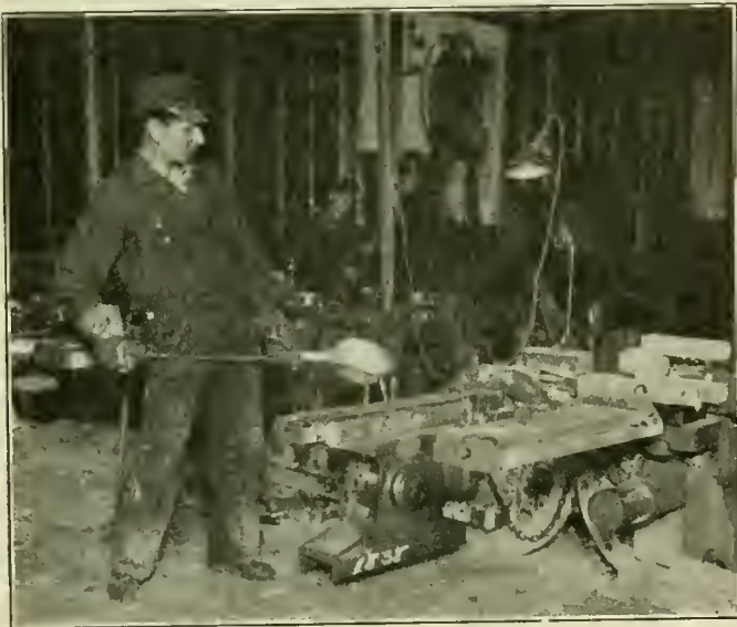
Fig. 2—Pouring Babbitt in Alligator Crosshead Gib
