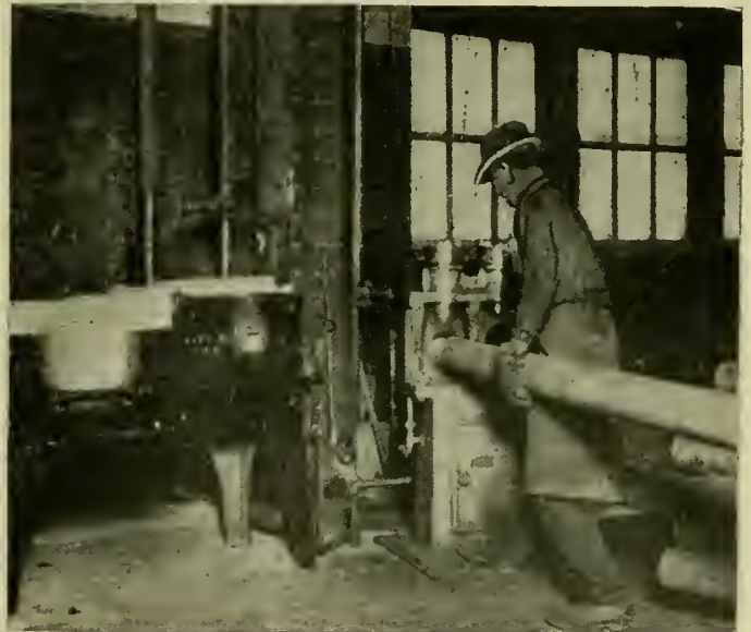
Fig. 9—As in the Case of Small Tubes the Superheater Flues Are Welded and Swedged on a Double Pneumatic Hammer Which Operates at 80 to 100 Lb. Pressure.
