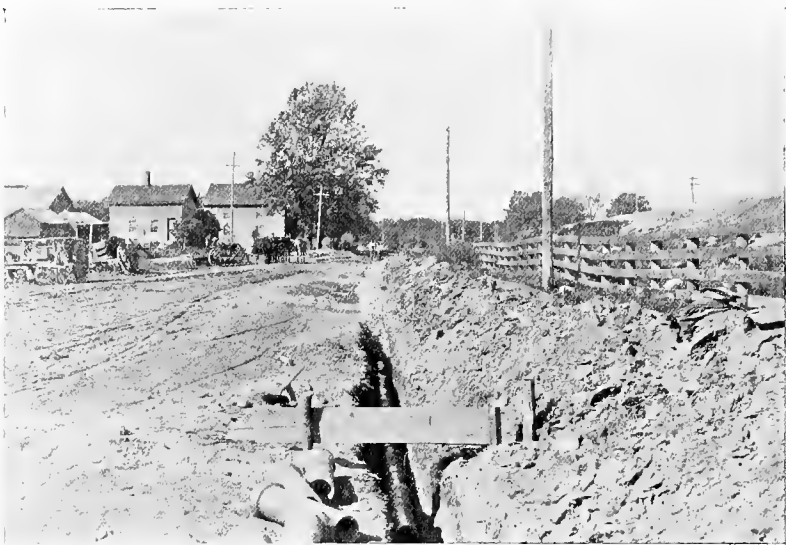
FIG. 7.—Laying side-drain for macadam road on state highway in Massachusetts.
