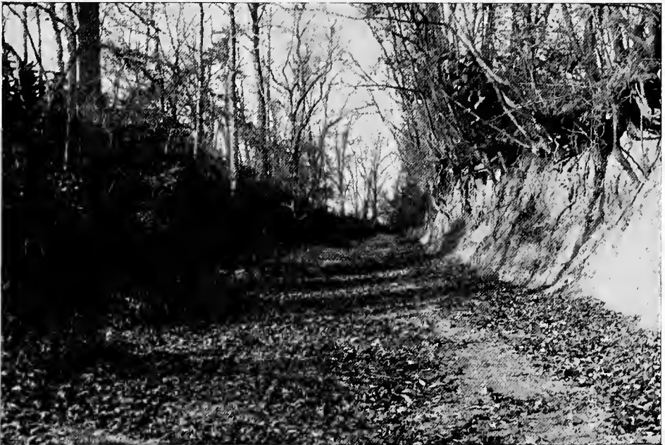
FIG. 2.—UNDRAINED ROAD IN CUT, CHARLES COUNTY.
