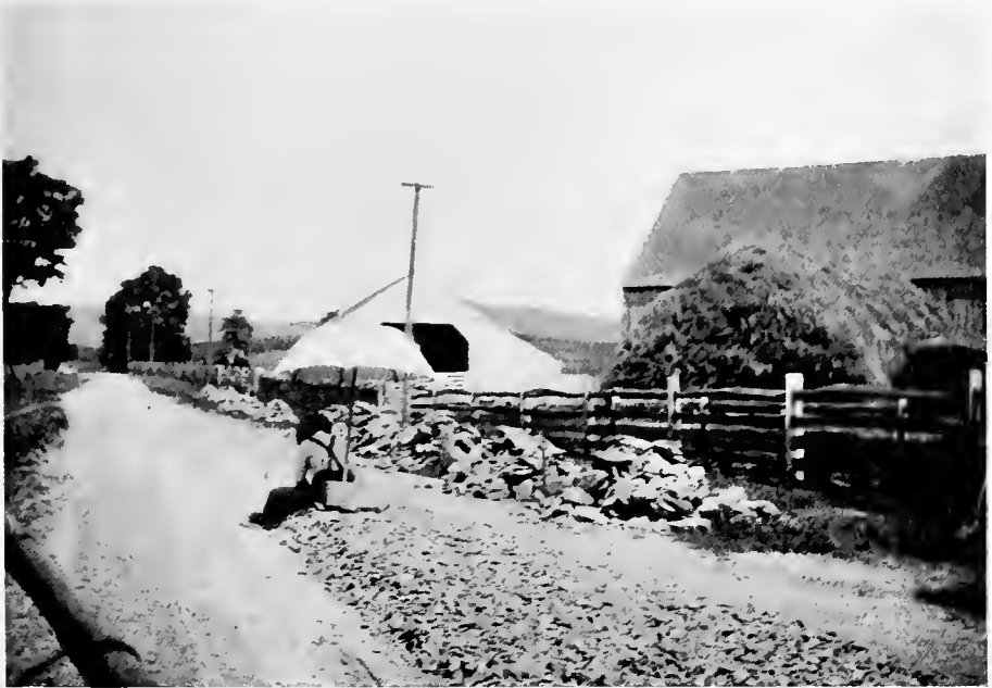
FIG. 1.—BREAKING STONE BY HAND, WASHINGTON COUNTY.
