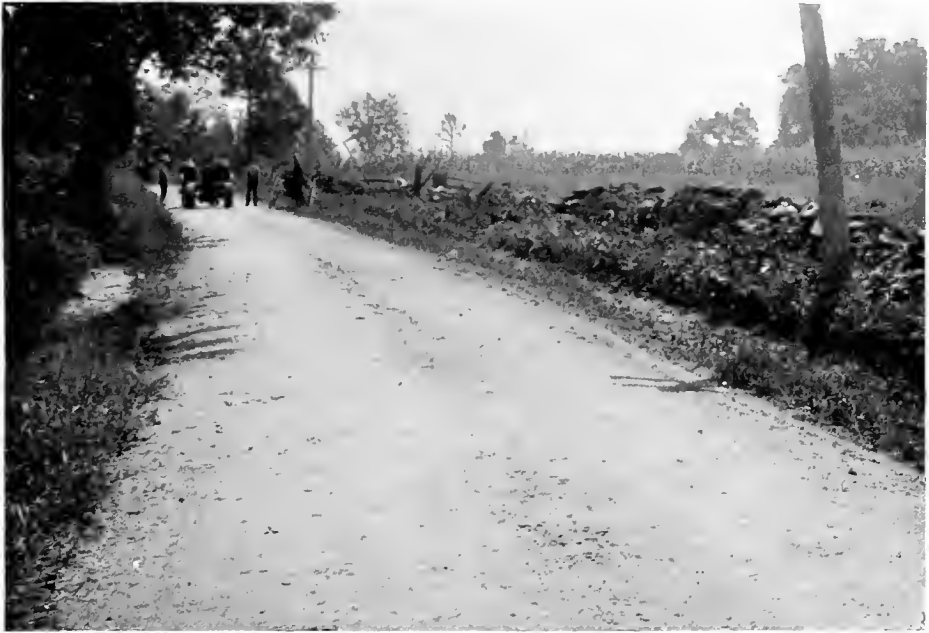
FIG. 1.—TRAP ROAD, BALTIMORE COUNTY. STONE SPREAD IN LAYERS AND ROLLED.
