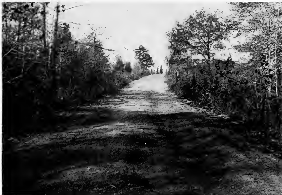
FIG. 1.—GRAVEL ROAD, PRINCE GEORGE'S COUNTY.
