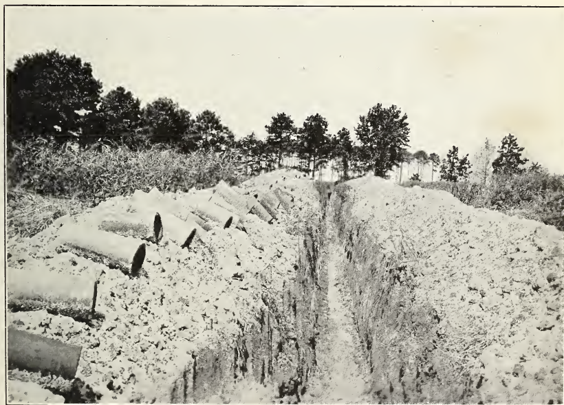
FIG. 2.—TILE DRAINAGE ON KEYPORT AND SUFFOLK FINE SANDY LOAMS, NEAR CHURCHLAND, VA.
