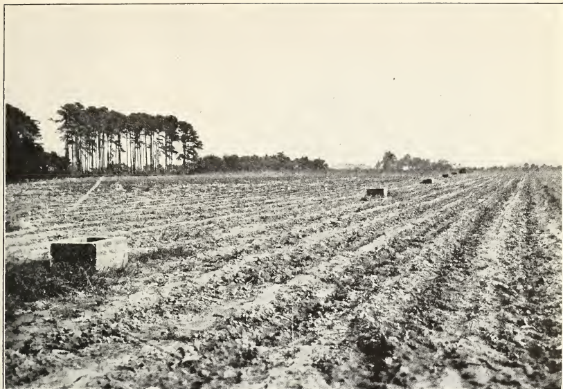
FIG. 1.—INTAKES FOR TILE DRAINAGE ON KEYPORT FINE SANDY LOAM, CHURCHLAND AREA, VA.
