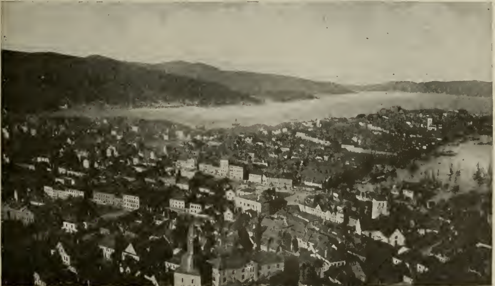
GENERAL VIEW OF THE HISTORIC TOWN OF BERGEN IN NORWAY
