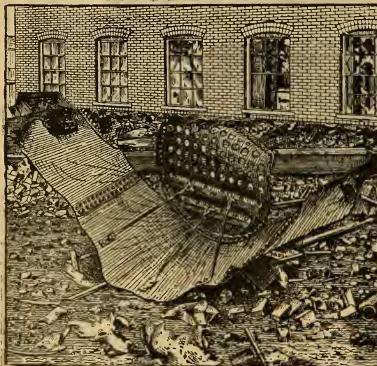
FIG. 3.—THE REAR END OF THE BOILER.
