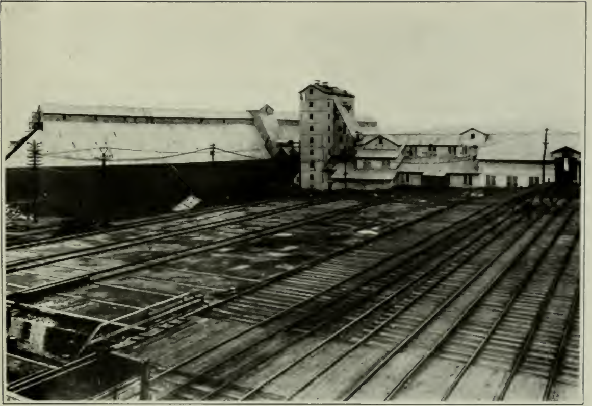
Asbestos Corporation of Canada, Ltd., King Mine at Thetford Mines, Que.—Railroad yard, crushing and drying plant, and 25,000 ton storage bin
