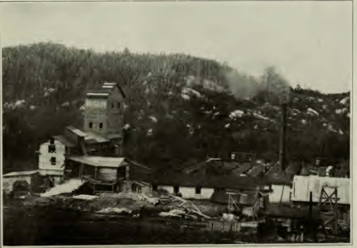
The Canadian China Clay Co. Ltd., St Remi, Amherst Township, Que.—Kaolin washing and Quartzite crushing plant.
