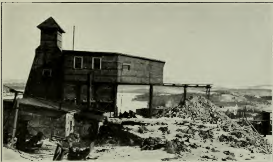
Mutual Chemical Co. of Canada, Ltd.,—Shafthouse at chrome mine on Lot 19 N. W., range X, township of Coleraine, Que.
