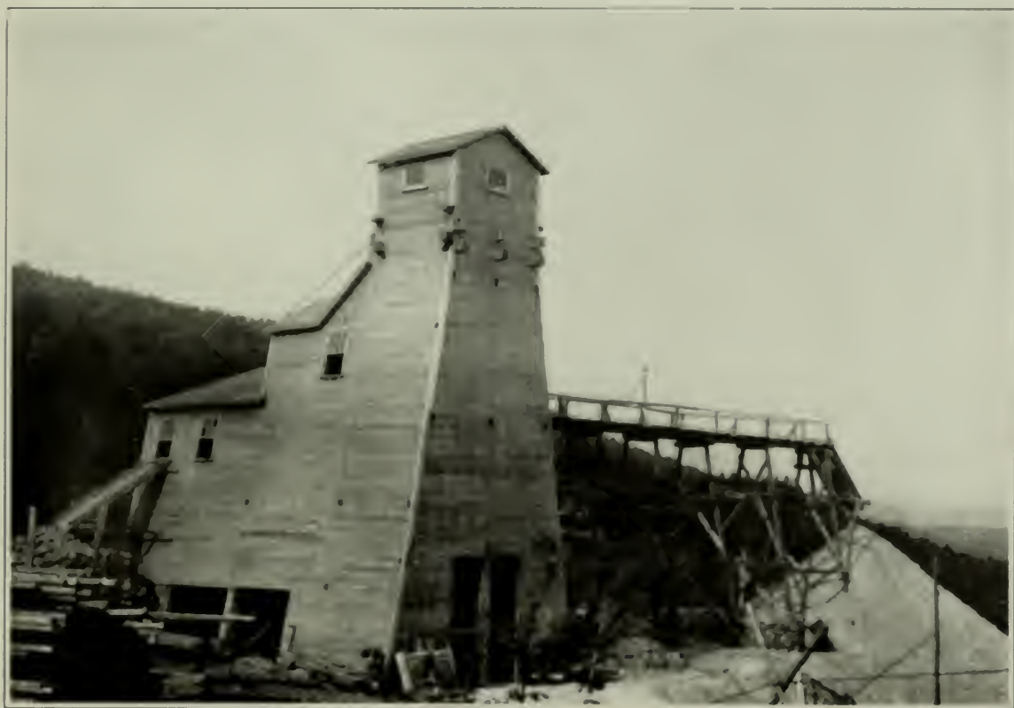
Black Lake Asbestos and Chrome Co. Ltd.,—Shafthouse at Caribou chrome mine block A, township of Coleraine, Que.
