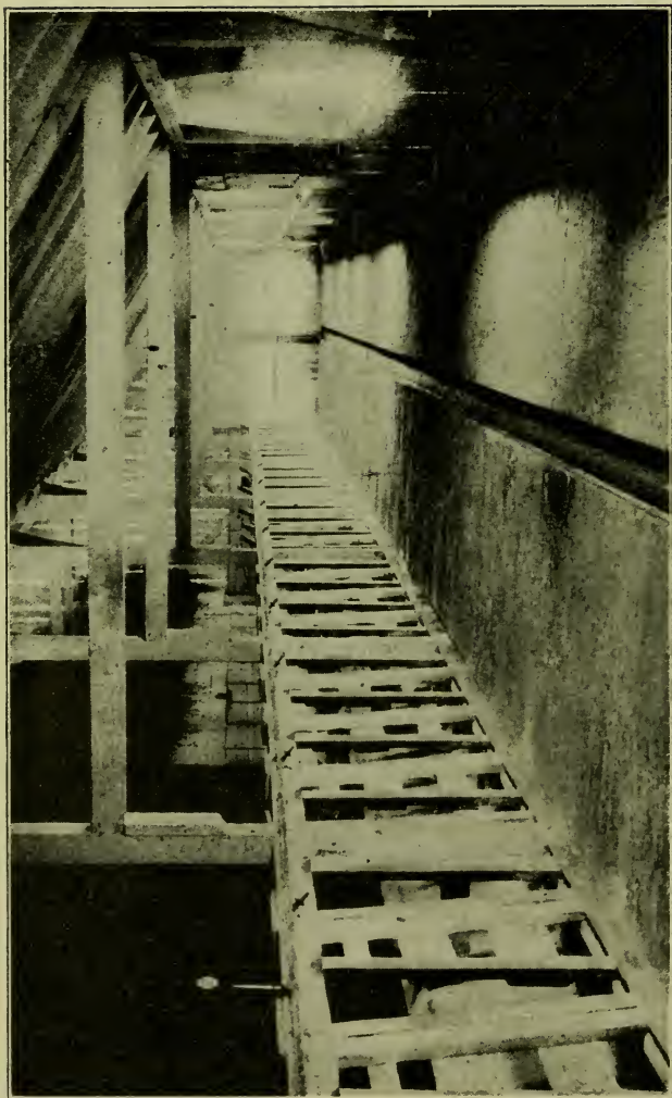
TYPICAL HUMBOLDT COUNTY COW BARN. INSIDE OF MR. JESS PETERSEN'S STABLE, NEAR LOLETA, CONSTRUCTED OF WOOD.
