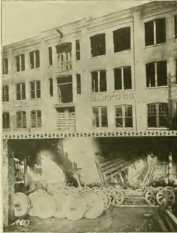
FIRE AT MCGUIRE SHOPS.
