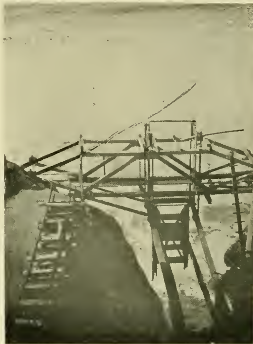
FIGURE 1. A WRECKED WAVE MOTOR.
