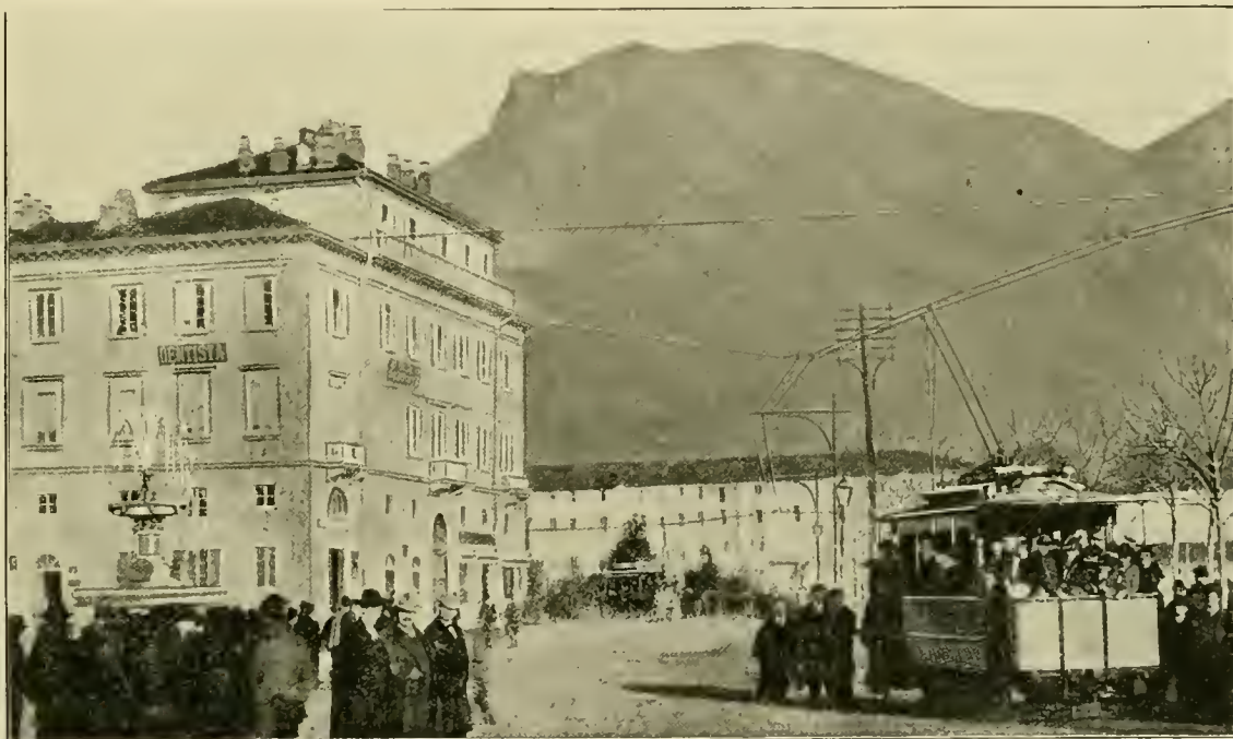
FIRST THREE PHASE ROAD IN THE WORLD, LUGANO, SWITZERLAND, DOUBLE TROLLEY AND GROUND RETURN.
