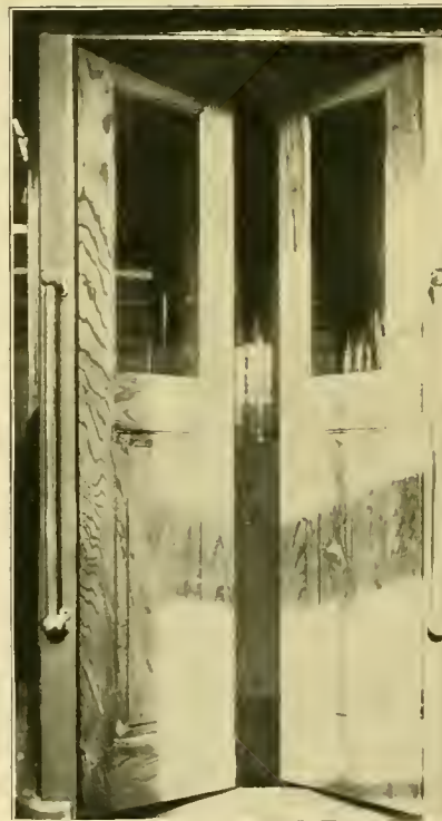
CALUMET VESTIBULE ON OLD CARS—DOORS SWING BOTH WAYS.
