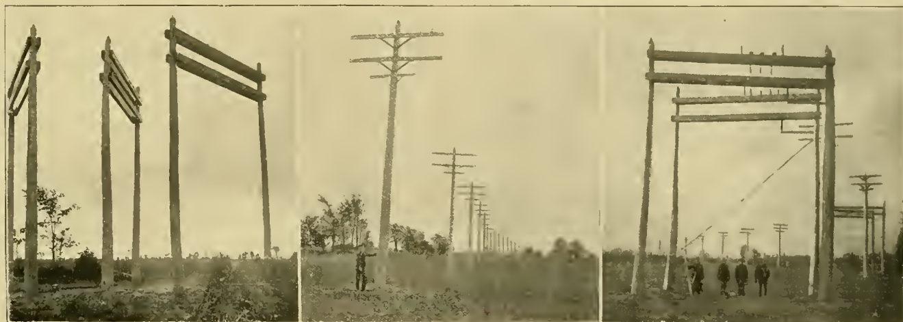
SAMPLES OF LINE CONSTRUCTION—NIAGARA FALLS-BUFFALO TRANSMISSION.
