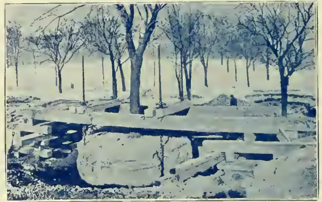
TREES RAISED TO ACCOMMODATE BOSTON SUBWAY UNDER BOSTON COMMON.
