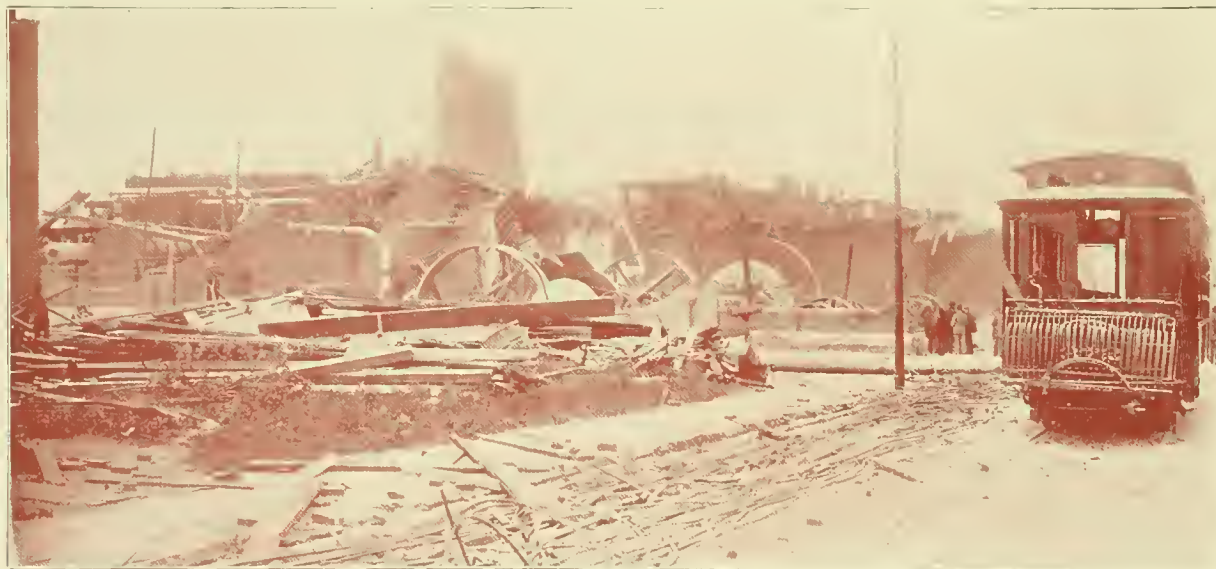
UNION DEPOT RAILROAD POWER PLANT AFTER THE CYCLONE.
