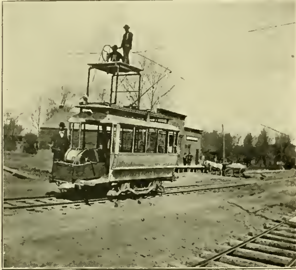
STRINGING LIVE TROLLEY WIRE—SIOUX CITY.
