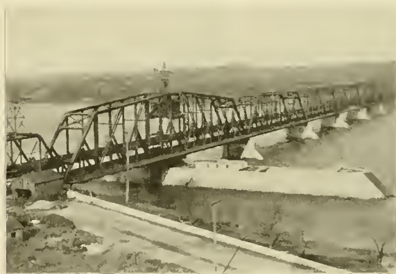
THE NEW ROCK ISLAND BRIDGE LOOKING WEST.
