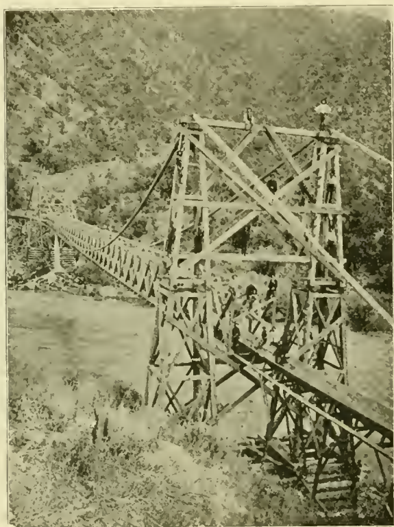
SUSPENSION BRIDGE FOR FLUME.
