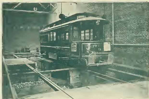
PITS AND CAR HOIST.
