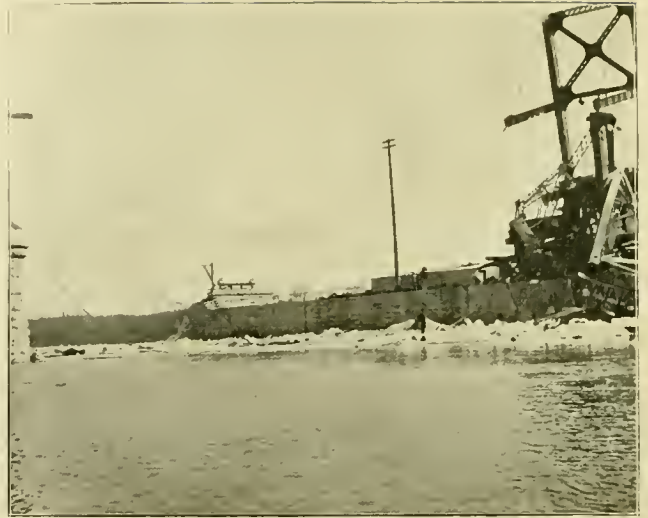
WRECK OF BRIDGE FROM DAVENPORT SIDE.
