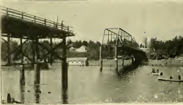
WRECK CLEARED AWAY.
