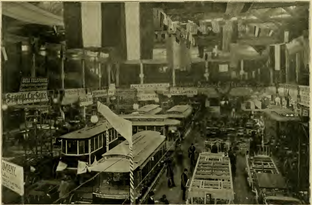
EXHIBIT HALL—LOOKING EAST.
