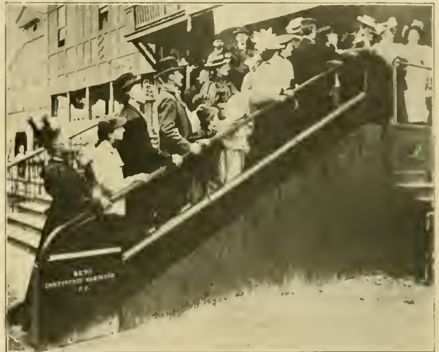
RENO INCLINED ELEVATOR AT CONEY ISLAND.
