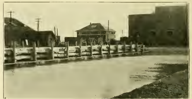
POND AND TROUGHS FOR COOLING CONDENSING WATER—CALUMET ELECTRIC RAILWAY, CHICAGO.
