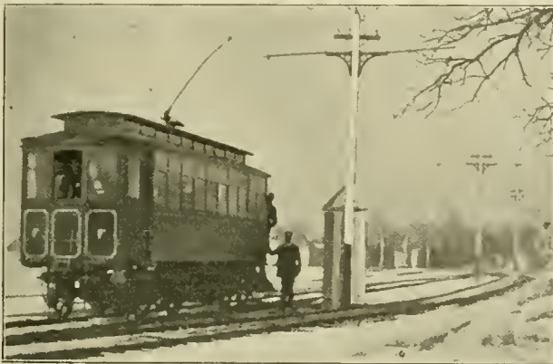
TELEPHONE BOX ON INTERURBAN LINE.
