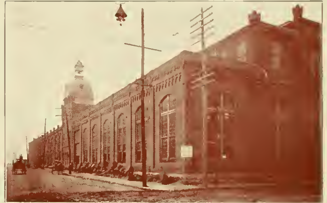
EXTERIOR ST. LOUIS IRON AND MACHINE WORKS.
