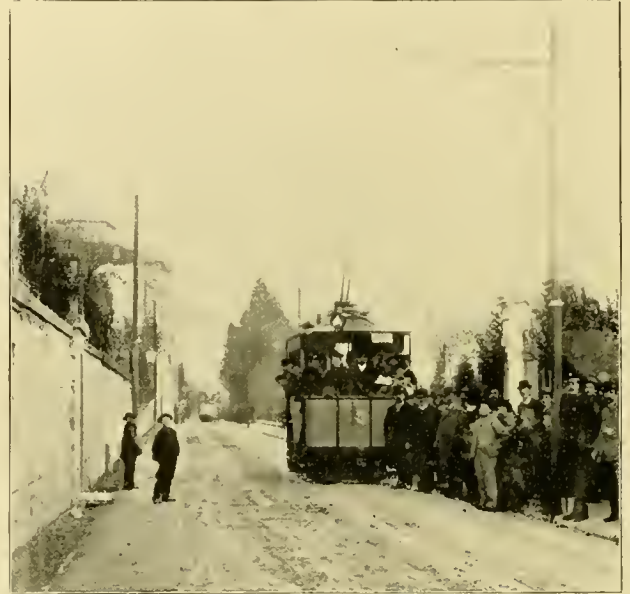
LUGANO—THREE PHASE ELECTRIC ROAD.
