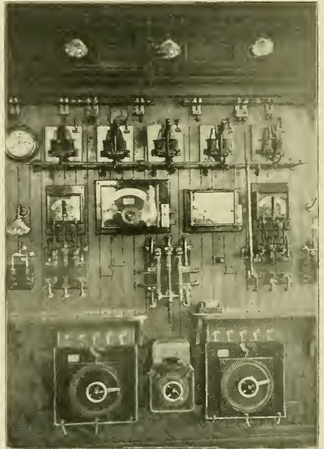
OLD WOODEN SWITCHBOARD.
