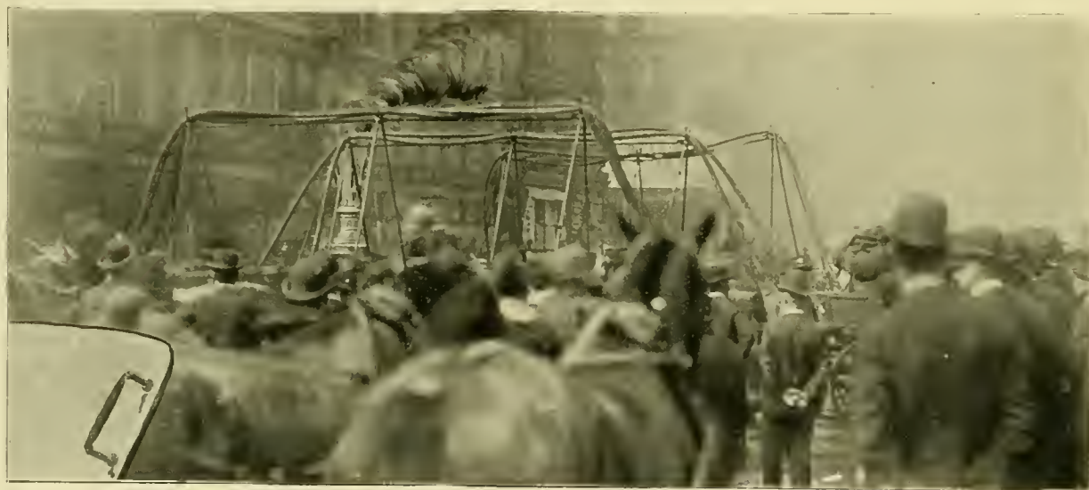
HOSE BRIDGES OVER STATE STREET, CHICAGO.
