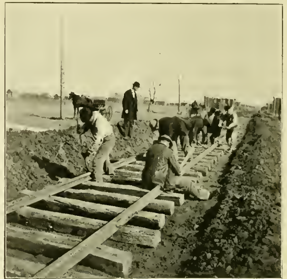
TRACK CONSTRUCTION AT SIOUX CITY.
