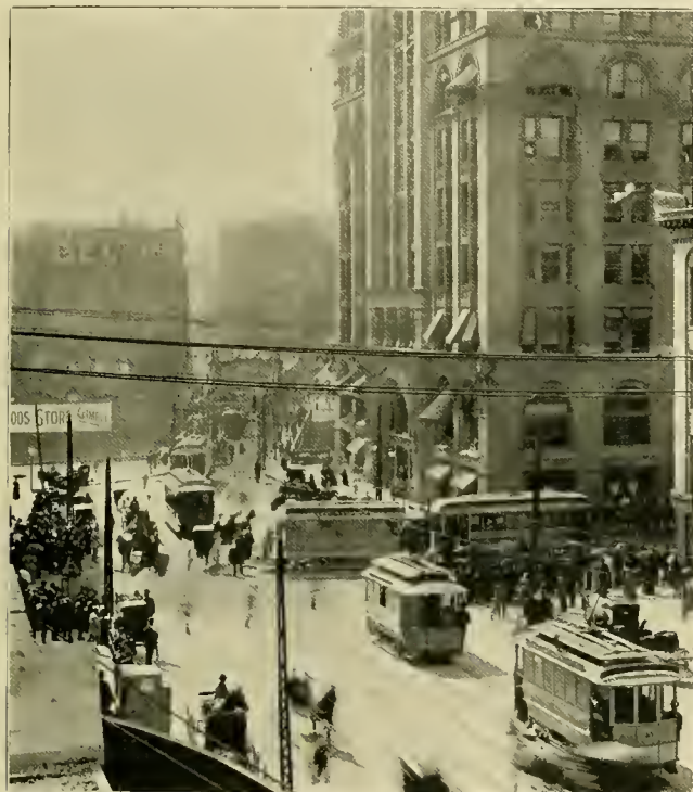
DERAILED TRAILER IN FRONT OF PFISTER BUILDING.
