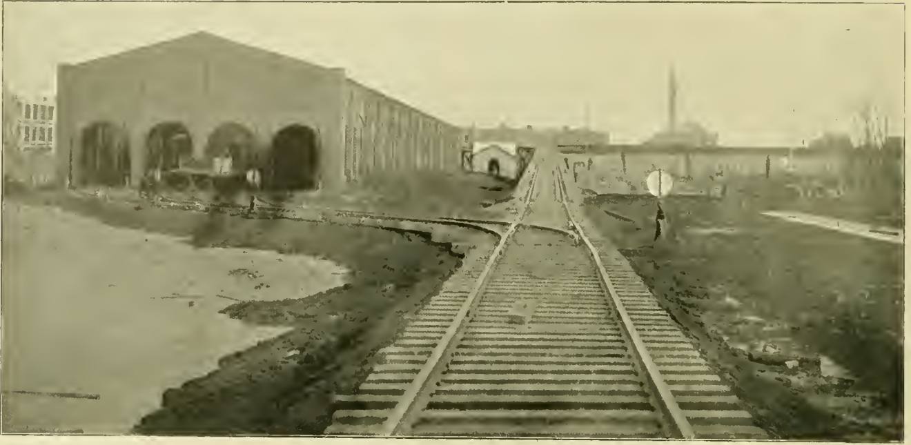
SHOPS AND INCLINE TO STRUCTURE—LAKE STREET, ELEVATED.
