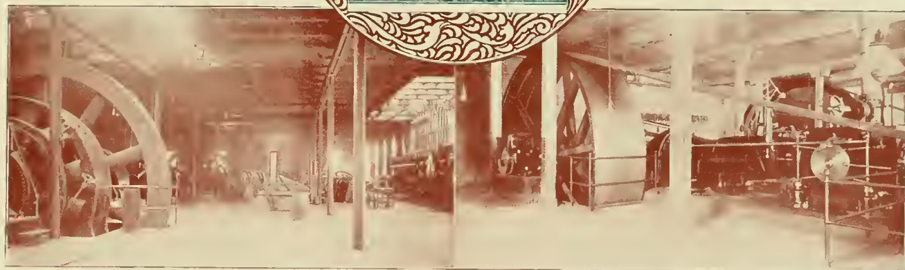
VIEWS IN UNION DEPOT POWER PLANT.
