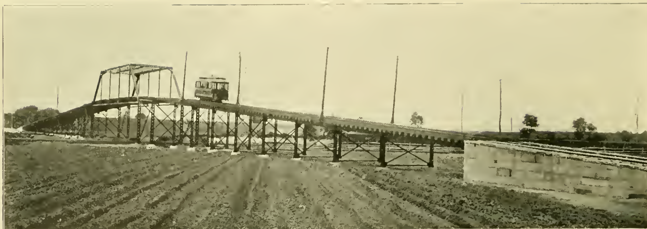
BALTIMORE, MIDDLE RIVER &amp; SPARROW'S POINT VIADUCT OVER WILMINGTON &amp; BALTIMORE RAILROAD.
