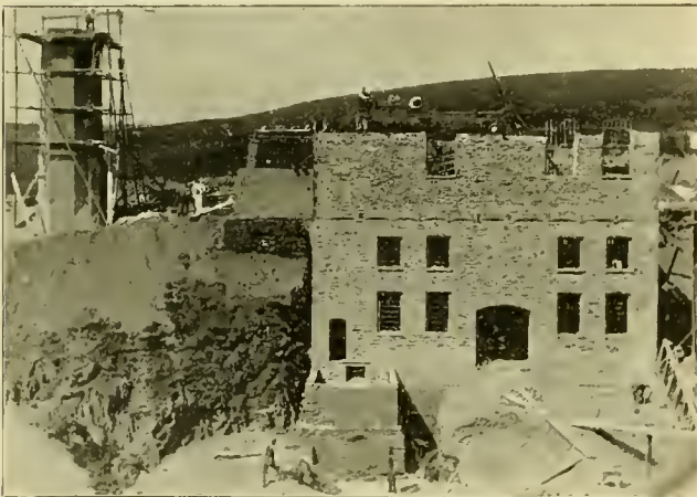
POWER HOUSE UNDER CONSTRUCTION, ISLE OF MAN.
