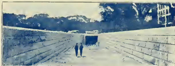
PUBLIC GARDEN ENTRANCE—BOSTON SUBWAY.
