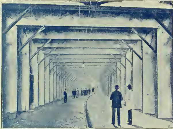
INTERIOR BOSTON SUBWAY.
