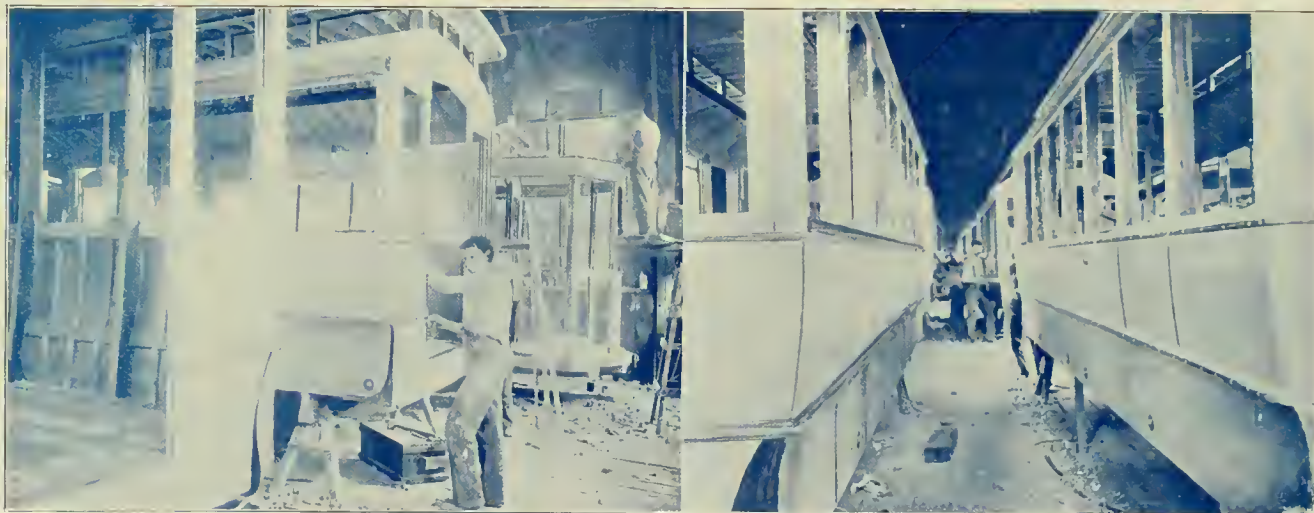
A GLIMPSE OF THE LACLEDE CAR COMPANY'S ERECTING SHOP.
