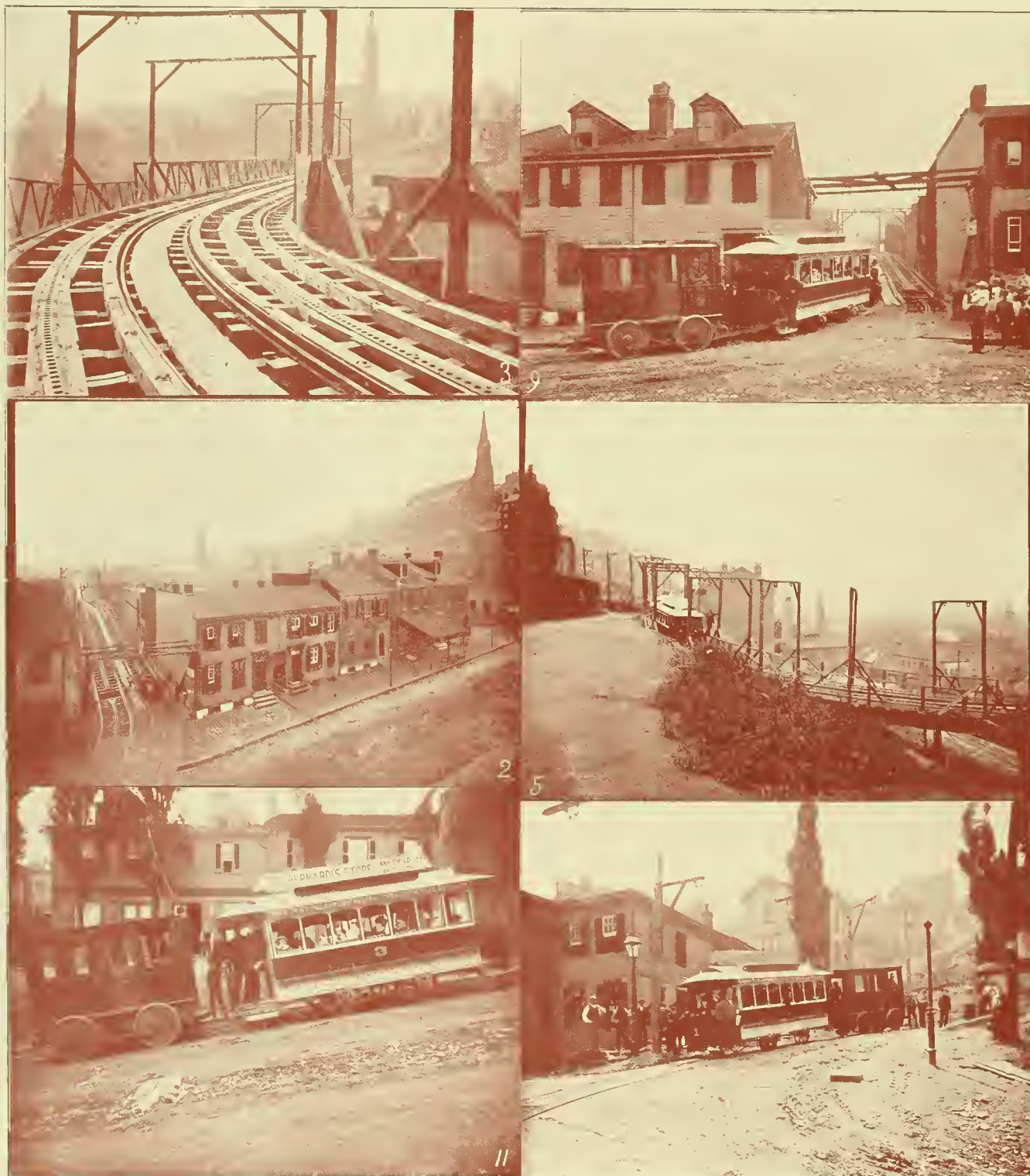
FIGURES 2, 3, 5, 8, 9 AND 11 SHOWING THE PITTSBURG, KNOXVILLE & ST. CLAIR RAILWAY — THE FIRST ELECTRIC ROAD IN PITTSBURGH — DAFT SYSTEM—OVER RUNNING TROLLEY.
