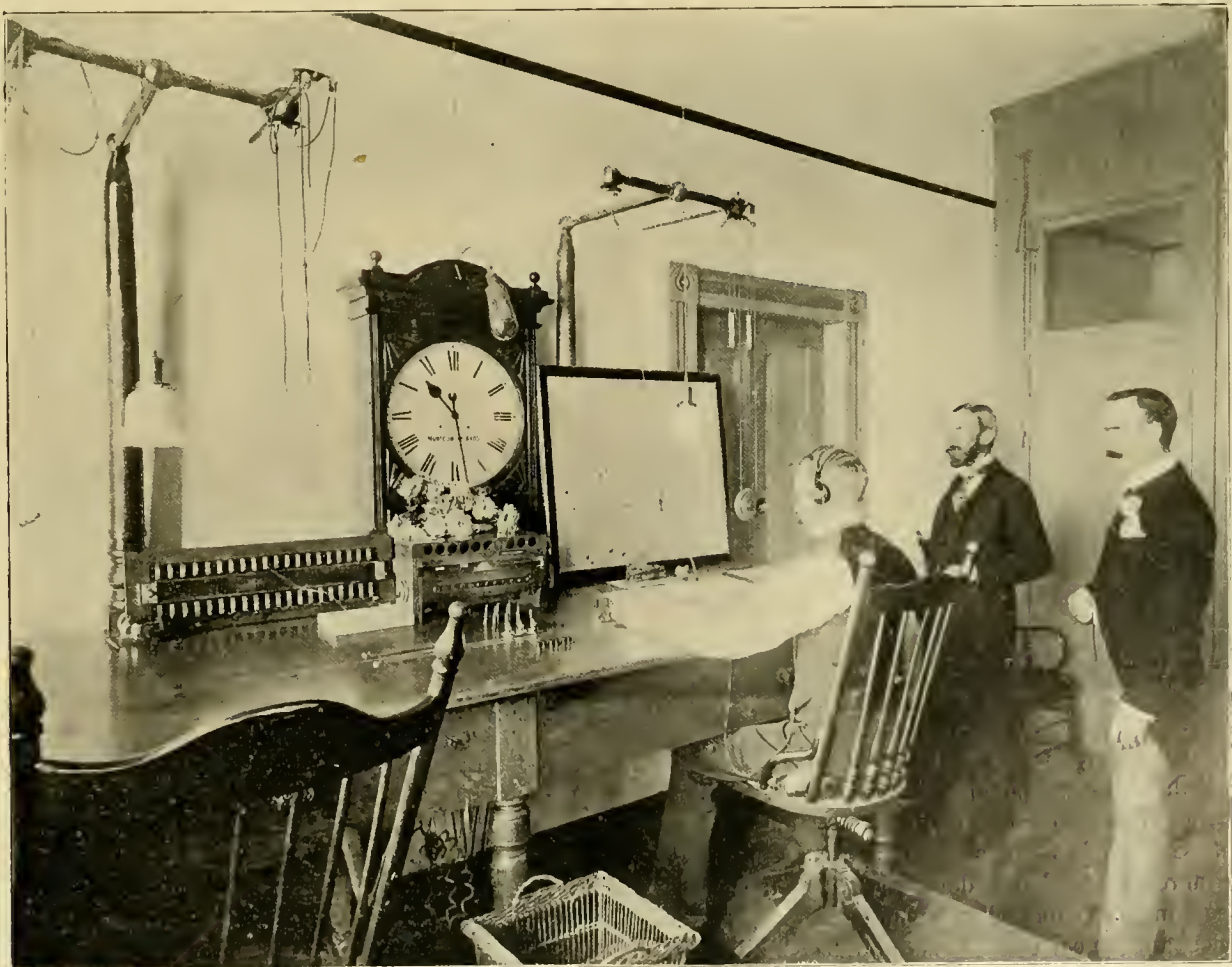
DISPATCHER'S OFFICE LOS ANGELES RAILWAY.
