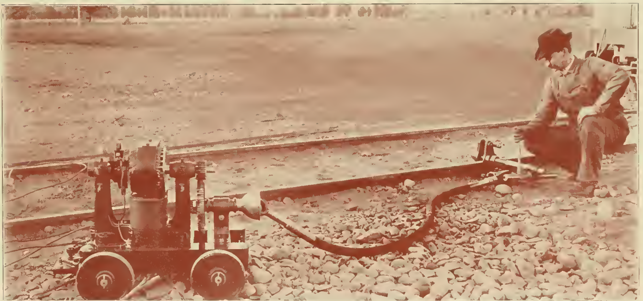
STOW TRACK DRILL IN OPERATION.
