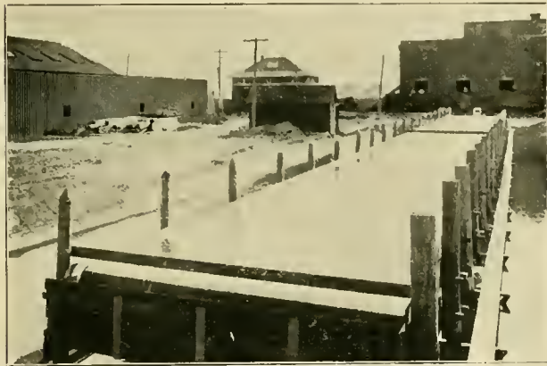
COOLING TROUGH FOR CONDENSING WATER-- CALUMET ELECTRIC RAILWAY, CHICAGO.
