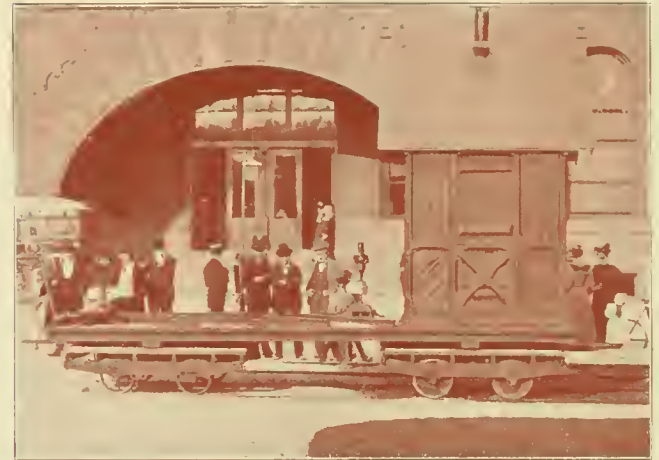
SWITCH YARD FLOAT.
