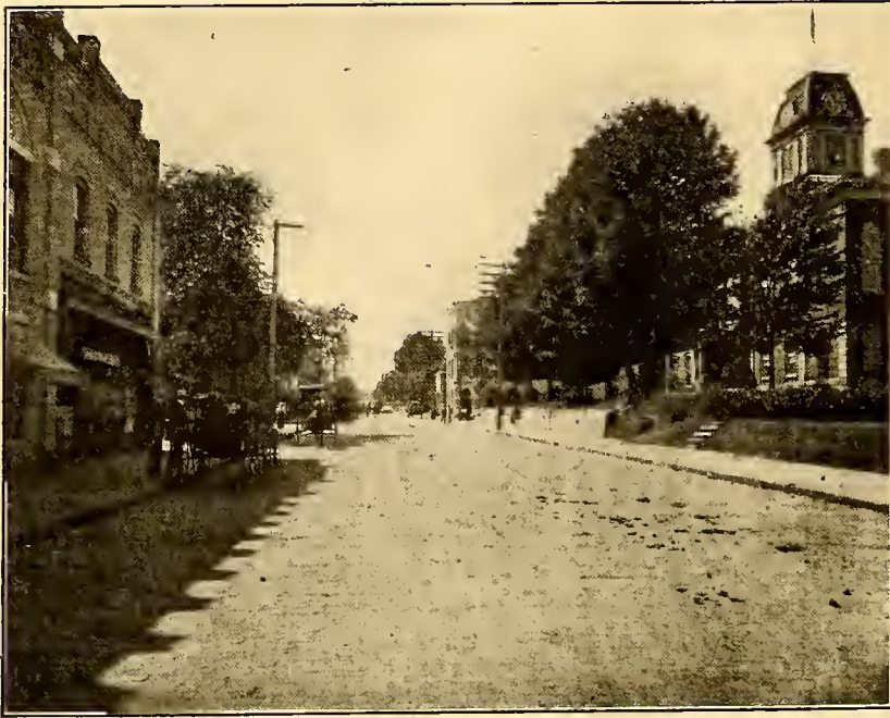
MAIN STREET OF WAYNESVILLE, HAYWOOD COUNTY.
