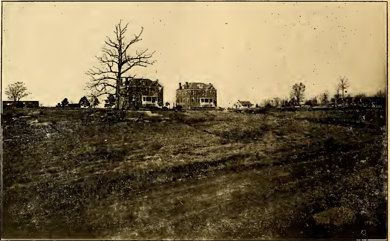
A BIRD'S VIEW OF BUILDING SITE.
