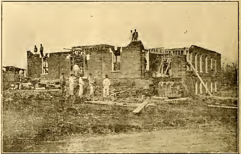
THE ADMINISTRATION BUILDING (UNDER CONSTRUCTION.)
