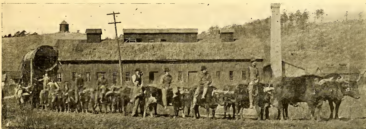
TEAM OF OXEN. AT SYLVA, JACKSON COUNTY, N. C., READY TO START 8 MILES ACROSS THE MOUNTAIN TO CULLOWHEE NORMAL SCHOOL, THE SPLENDID INSTITUTION ESTABLISHED BY PROF. R. L. MADISON IN THE HEART OF THE MOUNTAINS. THE BOILER WAS INSTALLED BY MR. B. MCKENZIE IN THE POWER HOUSE OF CULLOWHEE'S CENTRAL HEATING PLANT.
