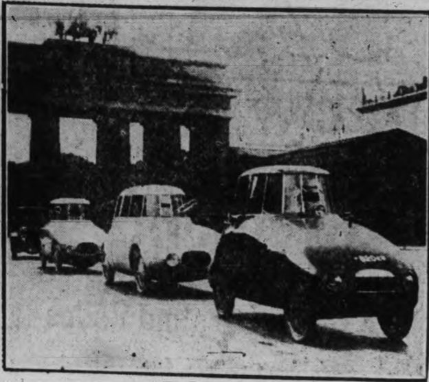
NEW TYPE OF AUTOMOBILE SEEN IN BERLIN. —The odd looking construction is supposed to give less resistance to the wind, and travels at a fair rate of speed. No running boards are seen, as the door of each side is the stepout. Forty to fifty miles are run on one gallon of gasoline.
