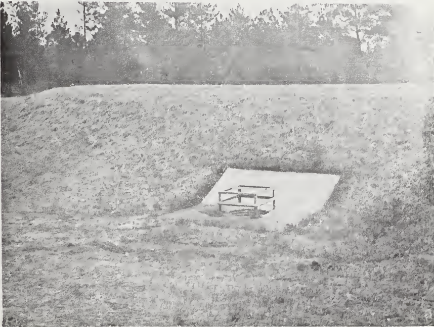
Same gully after treatment.
