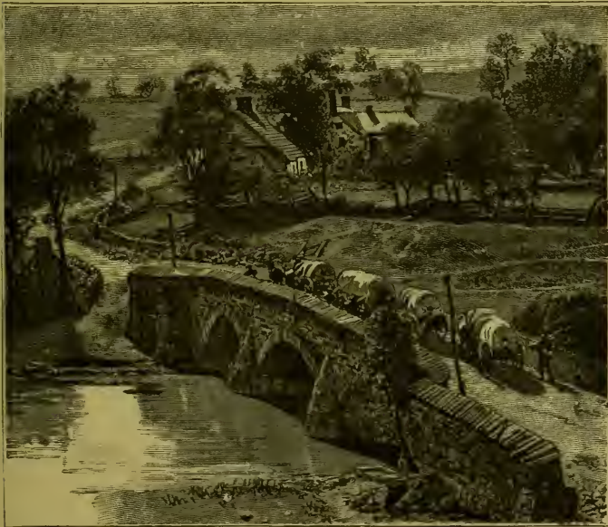
BRIDGE OVER THE ANTIETAM. 1
