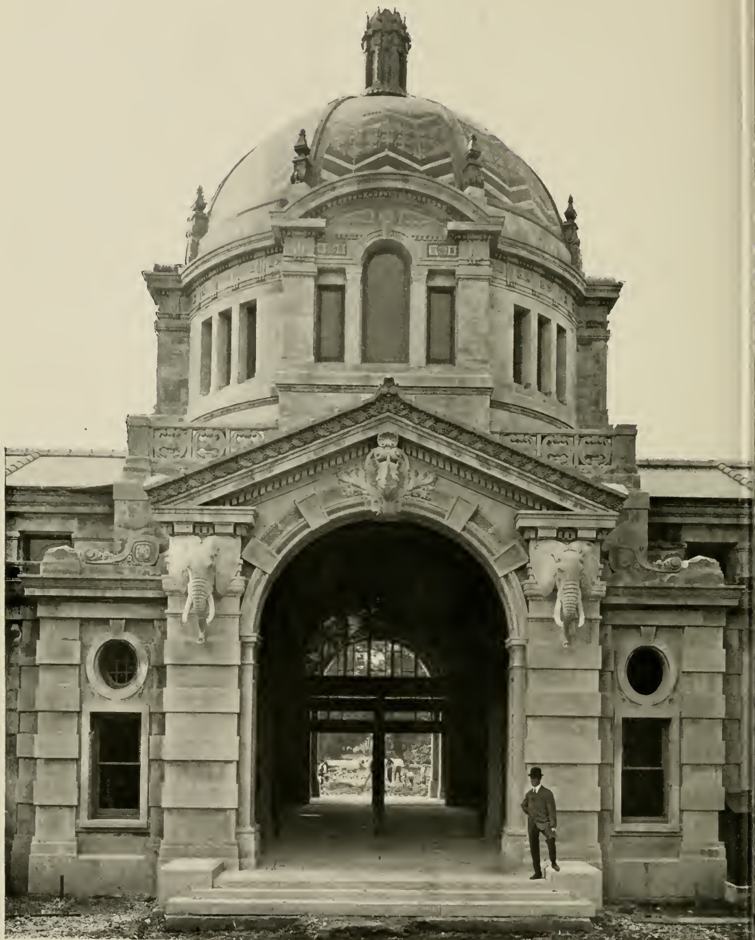
NORTH FACADE AND DOME OF THE ELEPHANT HOUSE. Heins & La Farge, Architects.
