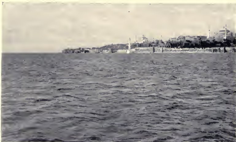
THE SOUTHEAST SEA WALL
