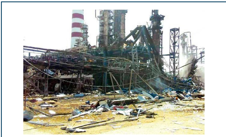
○ Fig. 1.7 Destruction of structures because of the accident at the Achinsk refinery in June 2014
