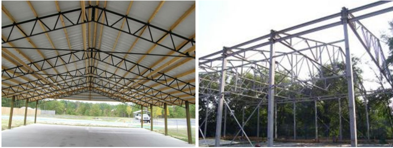
○ Fig. 1.3 General view of the steel truss
