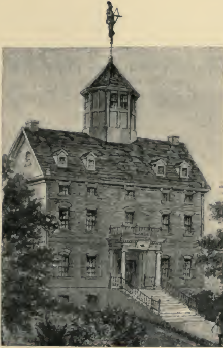
“The square front of the Province House, three stories high, and surmounted by a cupola, on the top of which a gilded Indian was discernible.”— Hawthorne's "Legends of the Province House."
