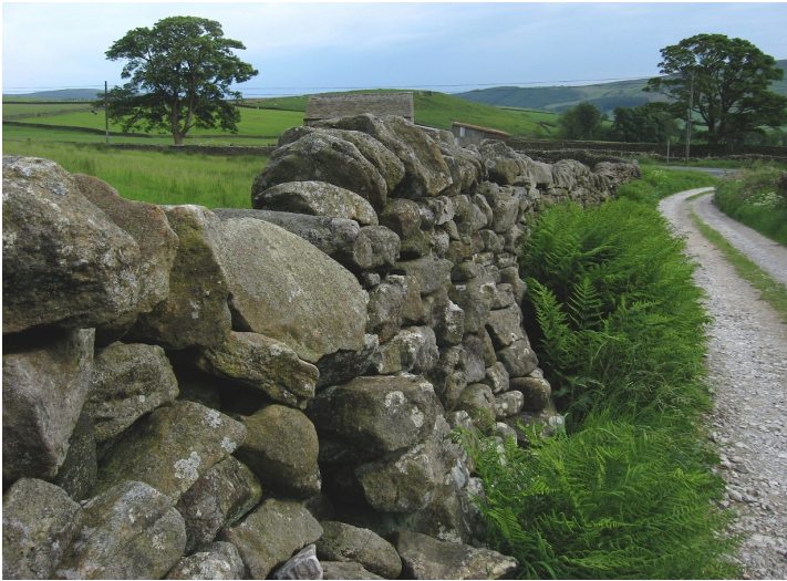
Figure 35 A dry-stone wall in England. Note how some stones stick out of the wall.
