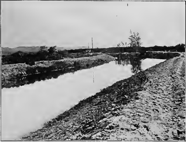
FIG. 52 b . Sunnyside Irrigation Canal, Washington
