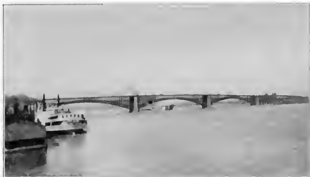
FIG. 29. Bridge across the Mississippi at St. Louis.
