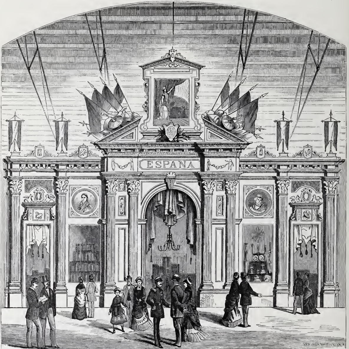
Main Building—Spanish Court.
