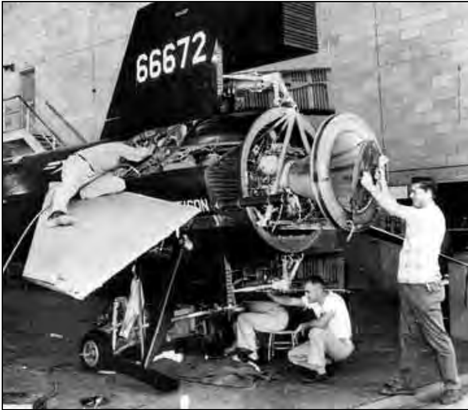
Technicians at the Flight Research Center work on the XLR99 engine. Note the corrugations on the aft end of the fuselage sponsons and vertical stabilizer. This was one of the keys to allowing the X-15 to withstand the high temperatures encountered during hypersonic flight. The blunt ends of the verticals and fuselage tunnels alone created as much drag as experienced by an F-104 fighter. (San Diego Aerospace Museum Collection)
