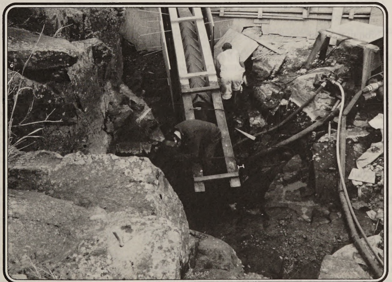
Construction of the Twentymile Creek Fishway.
