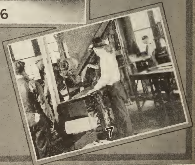
1—The mixing mill, mixing rubber and various compounds ready for calendering. 2—Cutting crude rubber into two-inch slabs for cracking machines. 3—Tearing rubber apart by hand for cracking machines. 4—Immense calender making side walls for cord tires. 5—Finishing Goodyear fabric tires. 6—Drying room. 7—Vertical bias cutting machine which cuts rubberized fabric into plies.
