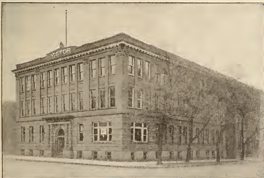
A fireproof building covering sixty thousand feet of floor space. It is here the various Victor Projectors are manufactured. The Victor plant is but one of many modern factories responsible for the rapid development of the city of Davenport, Ia.
